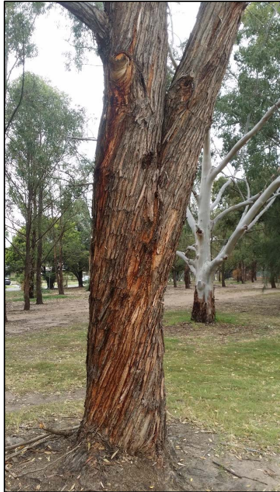
Plate 14 – showing weak junction on tree No. 65
