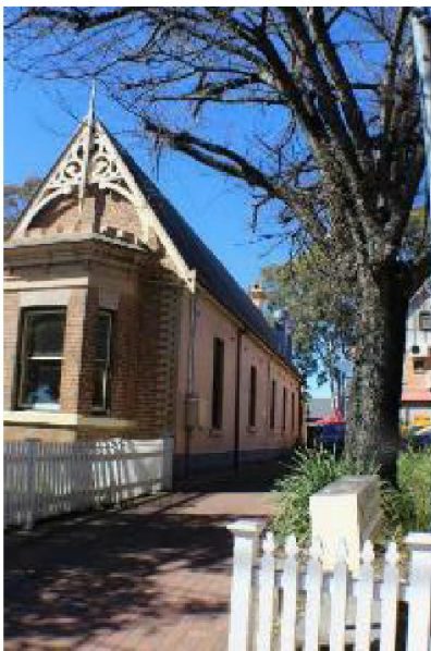
Figure 12: Driveway along western side of the building between 146 and 148 Station Street
