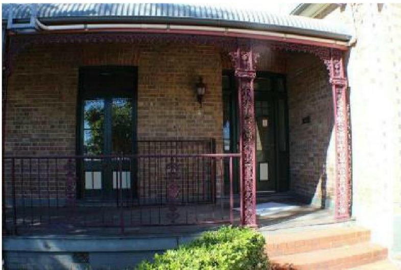
Figure 37: Reconstructed verandah with cast aluminum columns lacework
