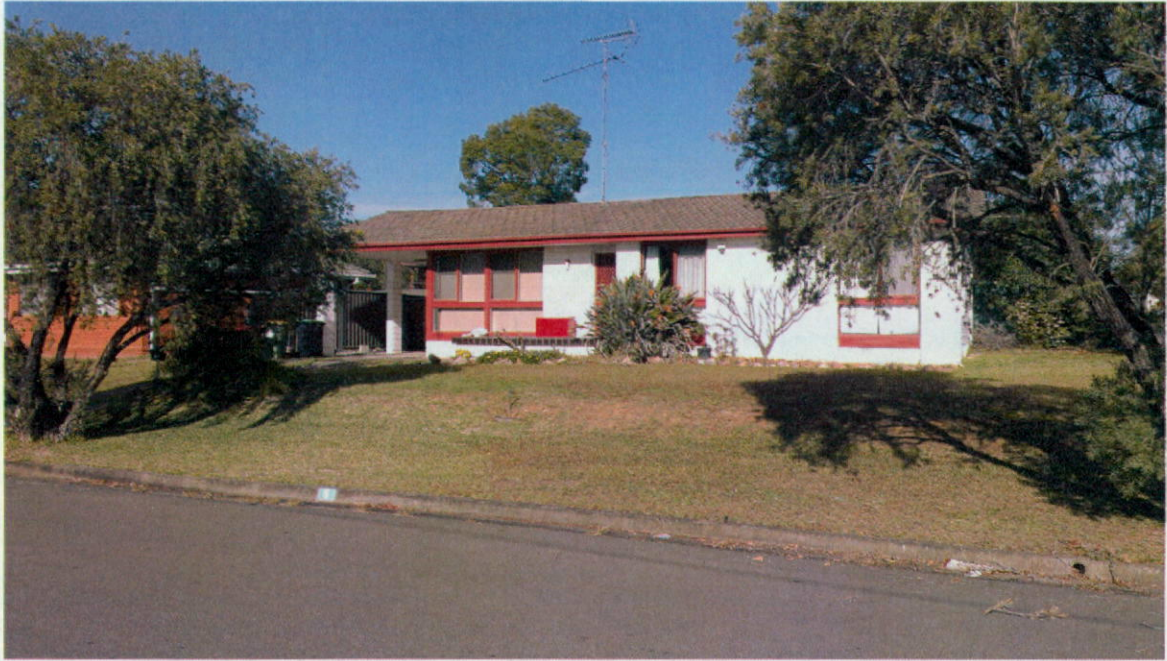
Above – Front view of existing house and site (as fronting Gamanya Avenue).
