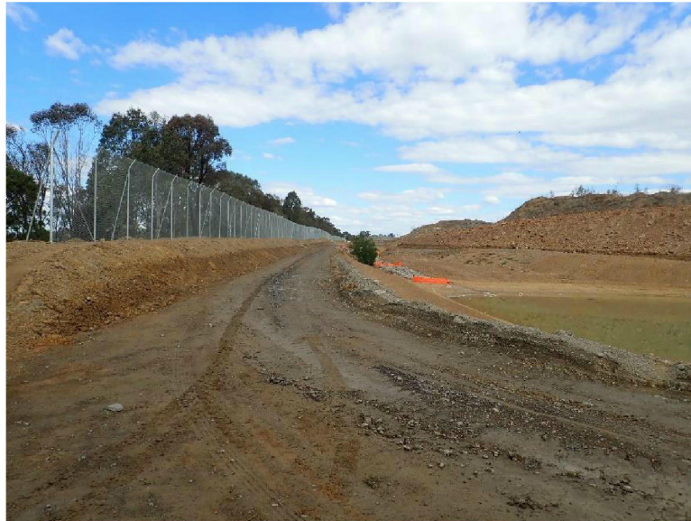
Photograph 07: View south along the access drive adjacent the eastern boundary.
