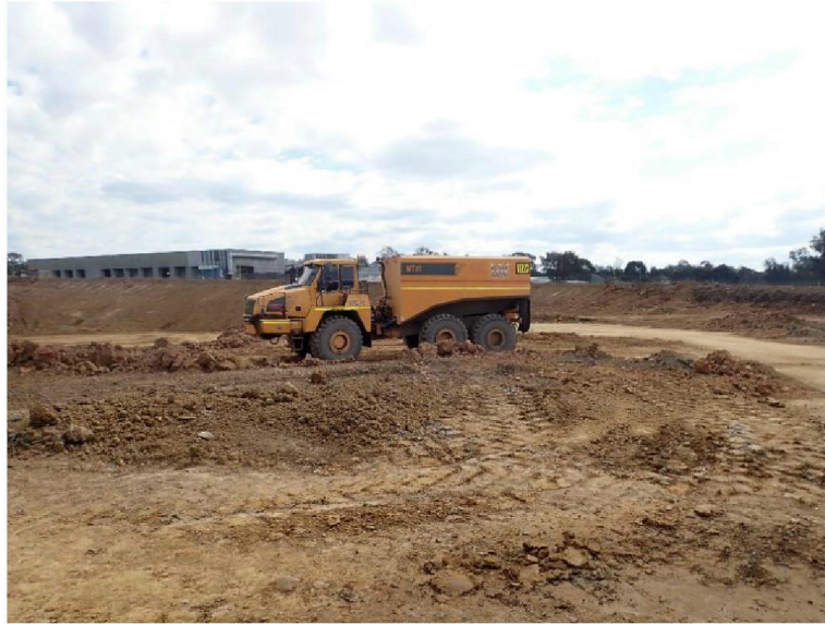
Photograph 09: 40 tonne CAT truck with spray bar and water cannon.
