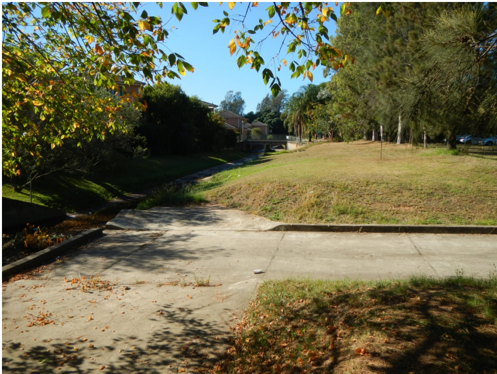
Photograph 5. View south east along concrete drain
