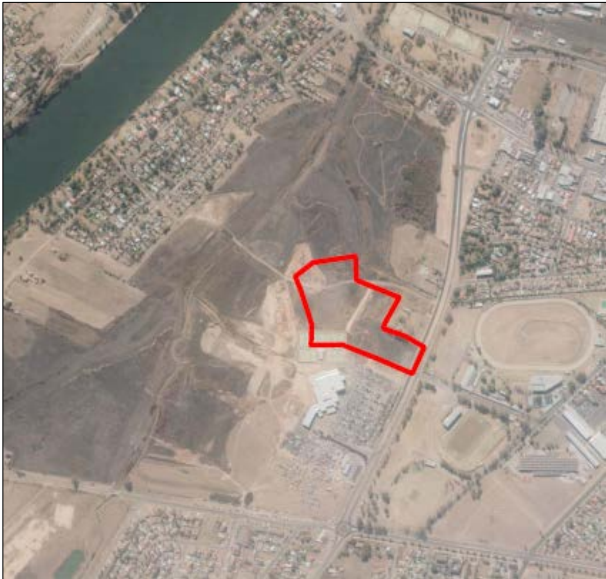
Figure 2. 1986 air photo showing extensive construction disturbance
