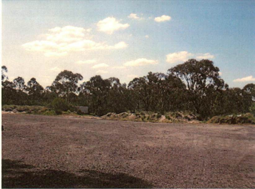
Rear turning area
