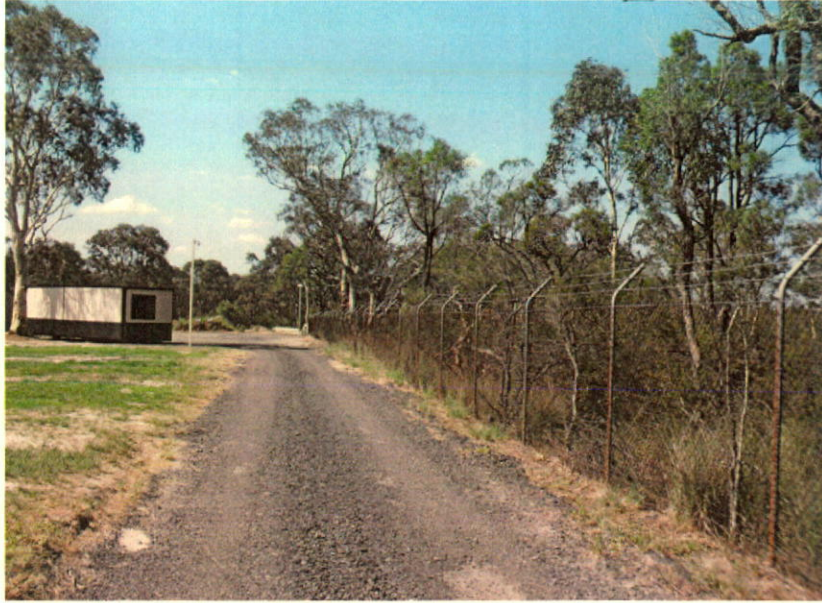
Showing the driveway looking towards the rear turning area
