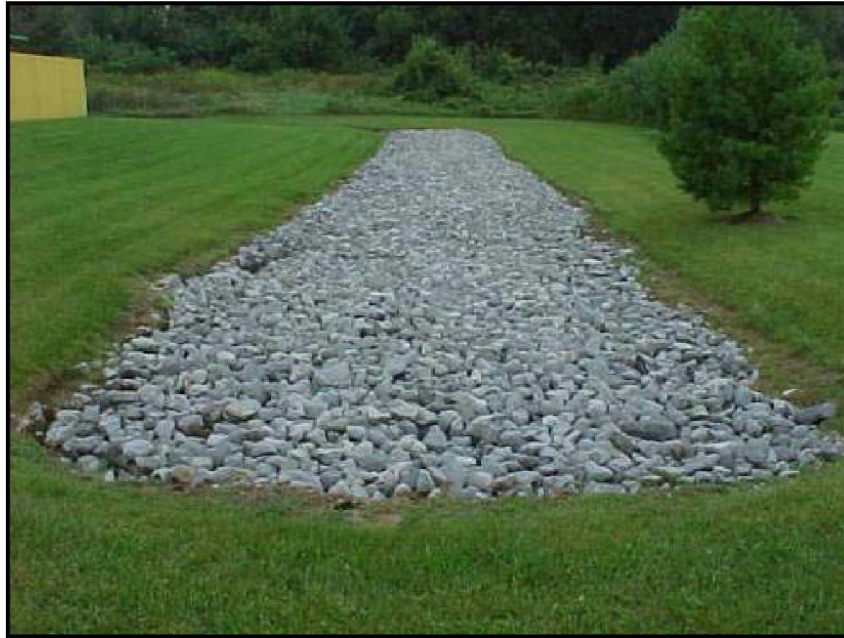
Plate 4.4 - Typical Infiltration Trench Arrangement
