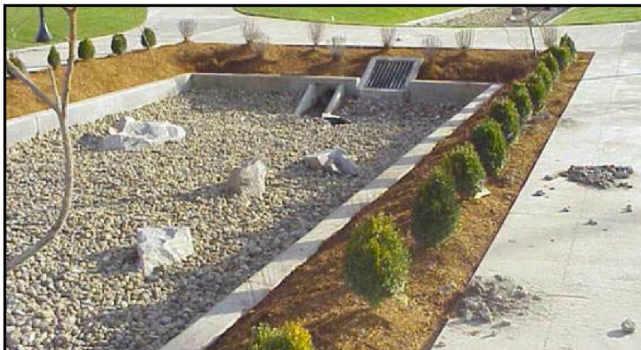
Plate 4.2 - Typical Sand Filter Arrangement
