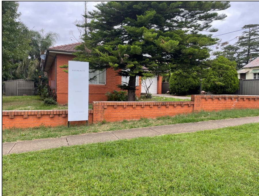
Figure 3: Photograph of 76 Hobart Street
