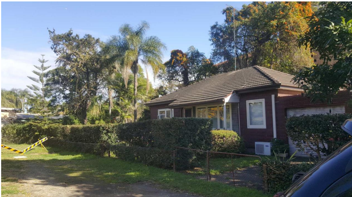
Figure 14 Photograph showing the existing dwelling and surrounding vegetation
