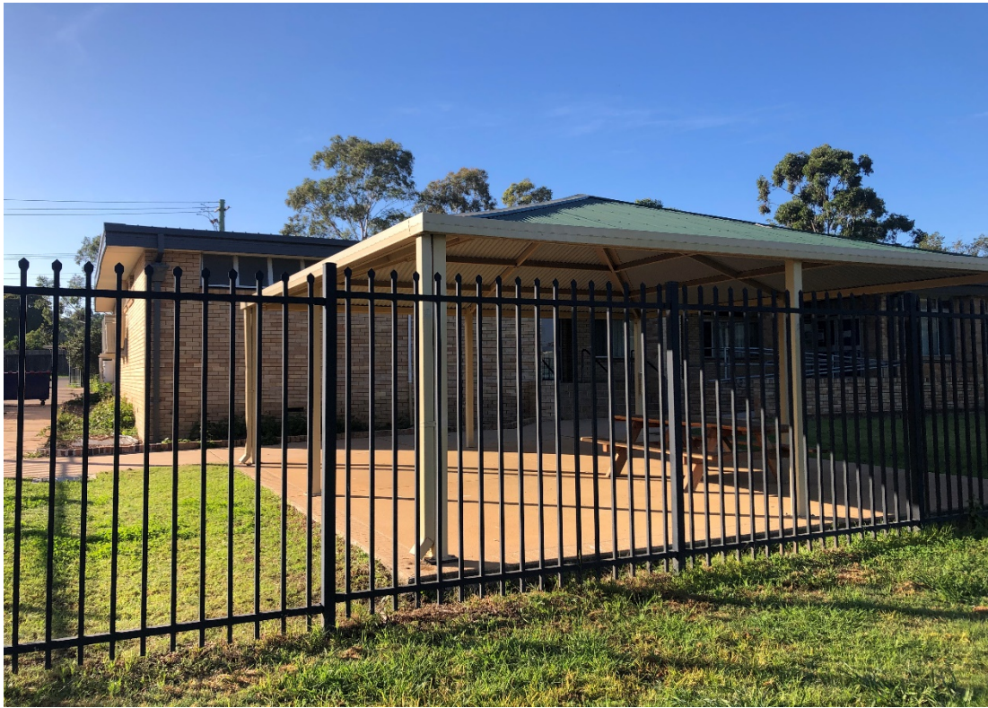
Photograph 6: Shows existing metal awning situated to the rear of the building
