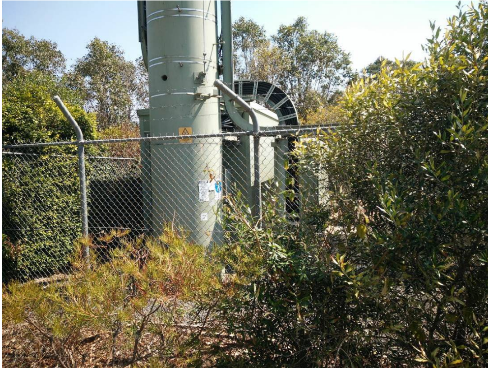
Photo 8 – Planted vegetation adjoining the communications tower
