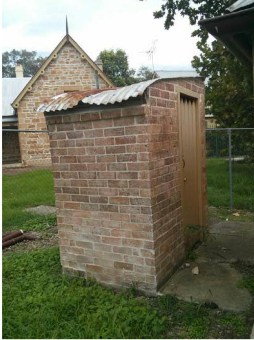
Former Emu Plains Public School toilet
