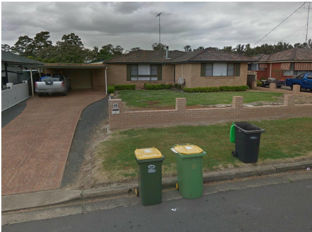
Photograph 1: Shows the subject site – 6 Edith Street, Kingswood
