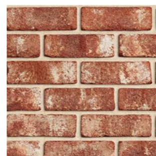
05 recycled brick external walls & subfloor
