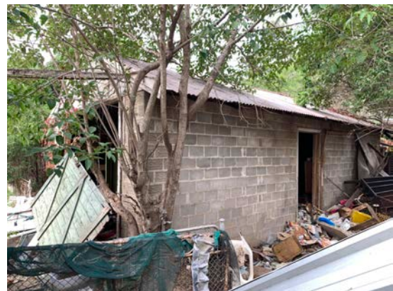
Figure 22: View of the detached garage structure.
