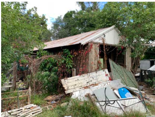
Figure 21: View of the detached garage structure.
