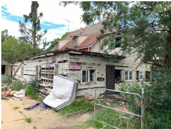
Figure 5: View of the northeastern elevation.
