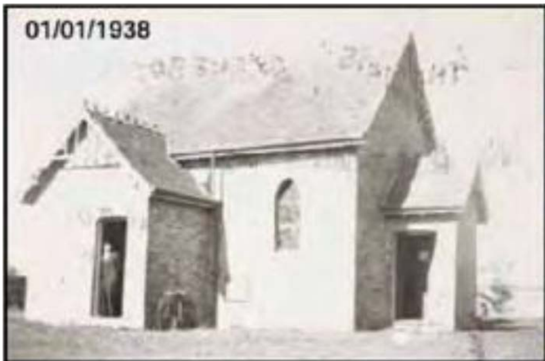
Figure 33: View of the former Holy Trinity Church in 1938.
