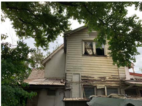
Figure 7: View of the southern elevation.
