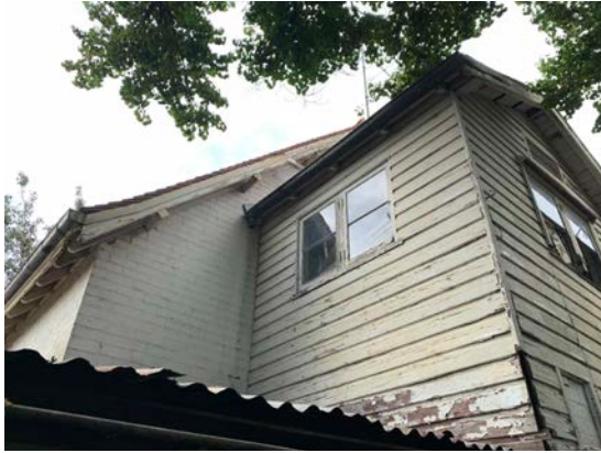
Figure 9: View of the southwestern elevation.
