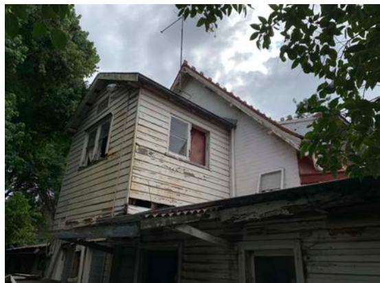
Figure 8: View of the southern elevation.
