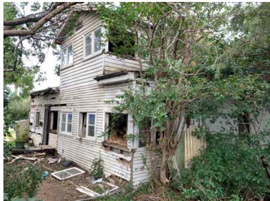
Figure 6: View of the northwestern elevation.
