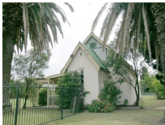
Figure 46: St Thomas' Anglican Church (former). [Source: NSW State Heritage Inventory, 2020]
