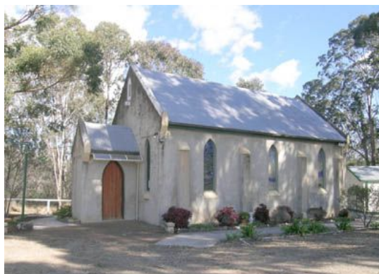
Figure 48: Luddenham Uniting Church. [Source: NSW State Heritage Inventory, 2020]
