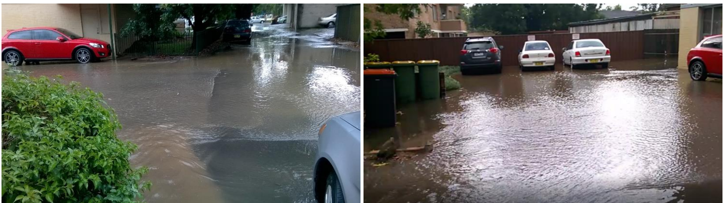
Figure 3-5 Flow from Station Lane to the back of 20 Union Road (Left) Station Lane looking toward Union Road (Right) Back of 20 Union Road Residence
