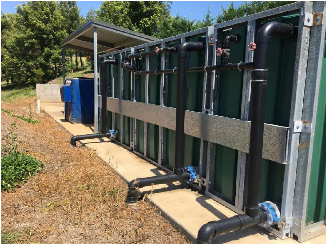
Photo 9 Example of treatment plant installed outdoors
