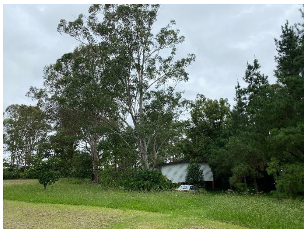
View of the rear elevation of the existing dwelling and trees to be removed
