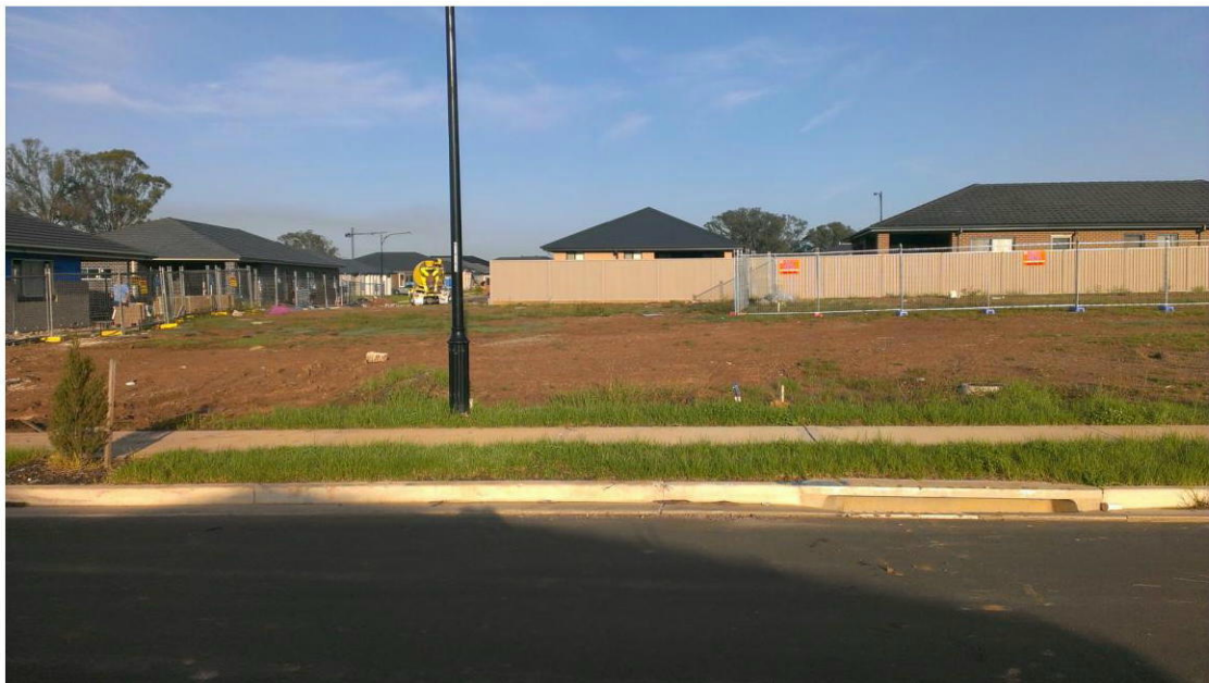
Below: View of site in-front of proposed Lot 2281B. Driveway access is OK and clear of light pole. Street tree will be relocated.
