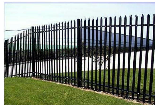
1800mm HIGH ALUMINIUM BLACK PALISADE SECURITY FENCE AND GATES
