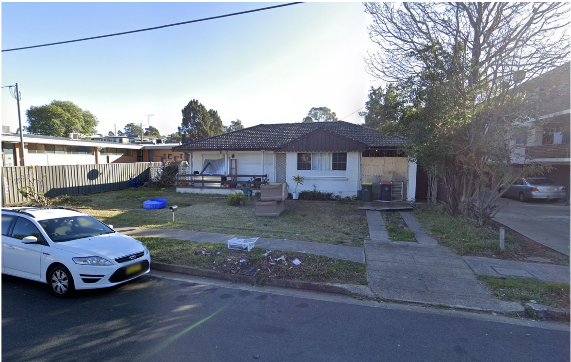
The subject property as viewed from Santley Crescent
