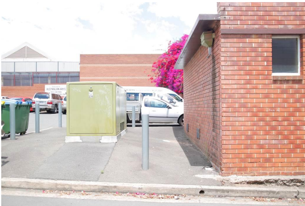
Figure 34: View of substation outbuilding and car park at rear of hotel
