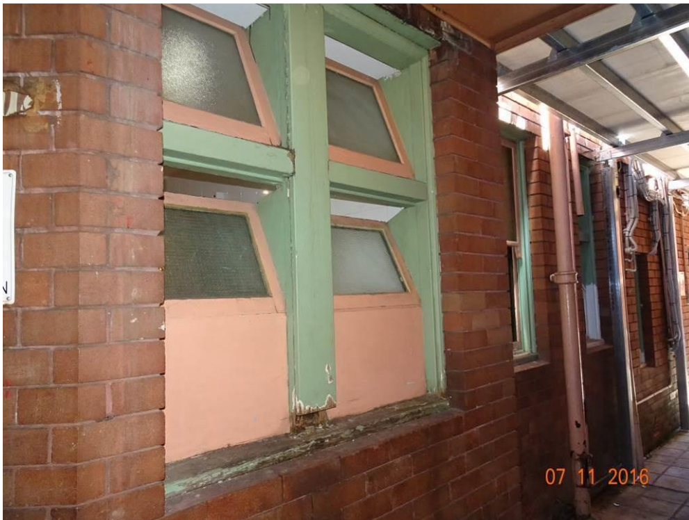
Figure 30: Ground Floor Eastern side showing windows to toilets and services pipework
