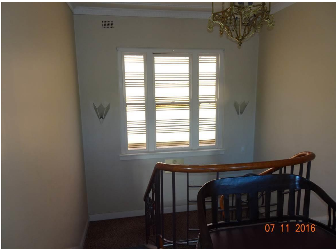
Figure 40: View of stair handrail, mid landing and window from First Floor
