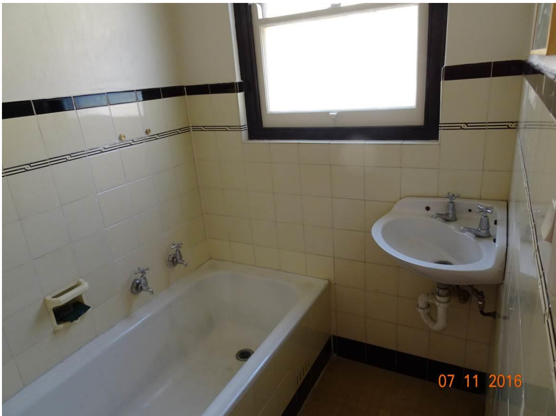
Figure 48: First Floor Ladies' Bathroom with original tiles
