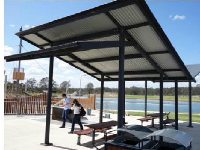
Shade shelters will encourage local group and family use for passive recreation.
