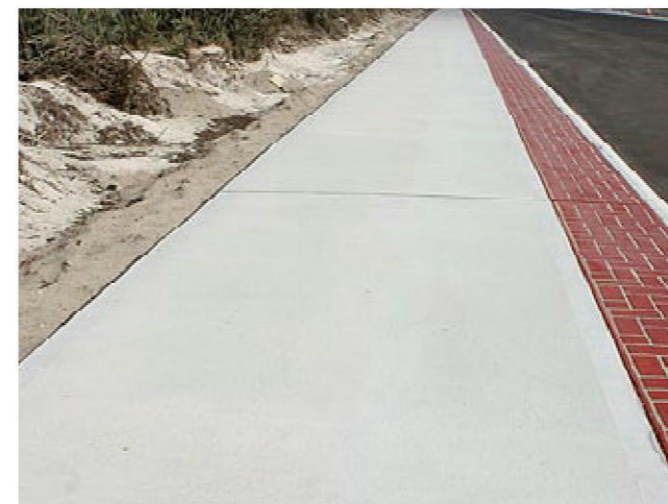
Broom finished concrete shared user path
