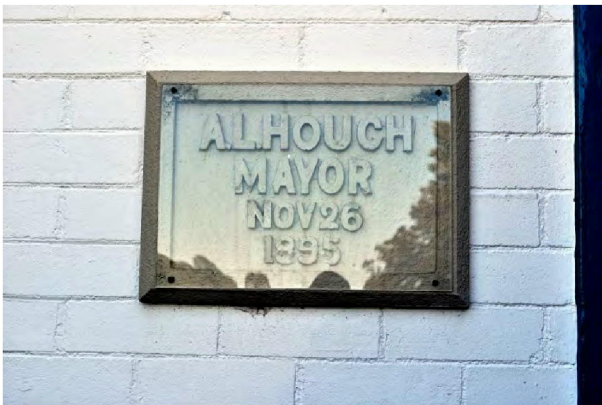
3. Foundation plaque to front wall- original building.
