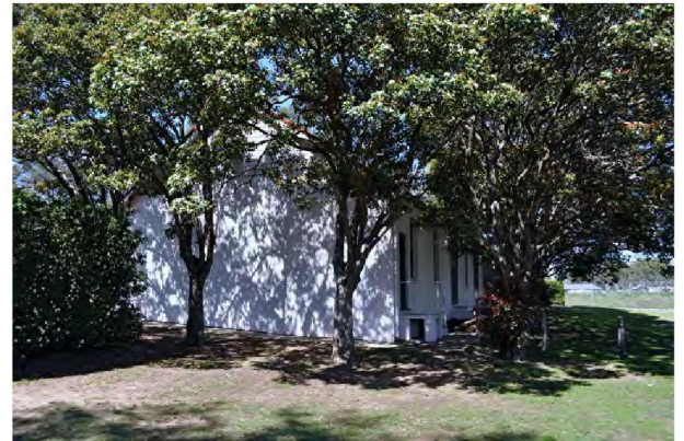
11. Rear (west wall).
