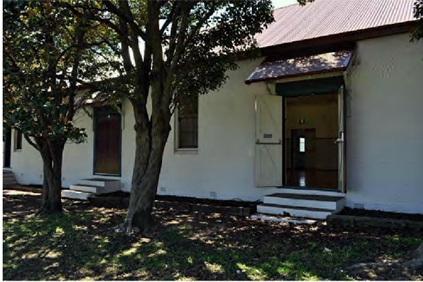
8. South wall- existing escape doors and steps.
