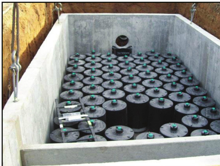
Plate 5.1 - Typical Cartridges Filter System (During Construction)
