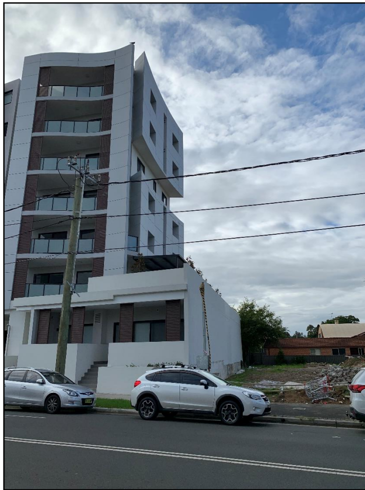
Photograph 3: View of the north-eastern side of the site looking from Station Street and showing the adjoining seven (7) storey residential flat building built to the common boundary at the ground floor level.
