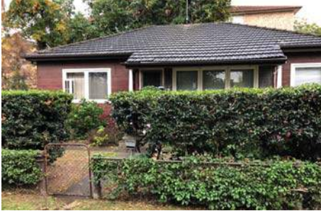
View of the front of the site Looking northwest Inspected 05.06.2018
