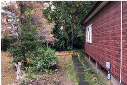
View of the southern side of the property Looking west Inspected 05.06.2018
