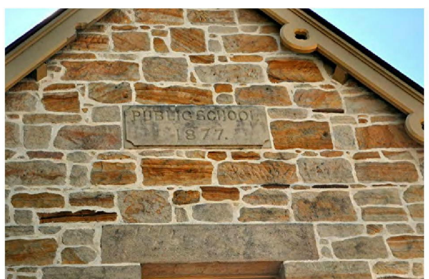
5. Name/ date stone to gable.
