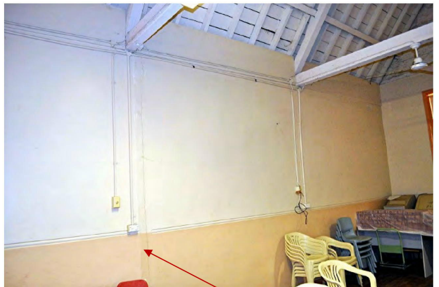
26. Surface-run conduits- schoolroom. Partition marking.
