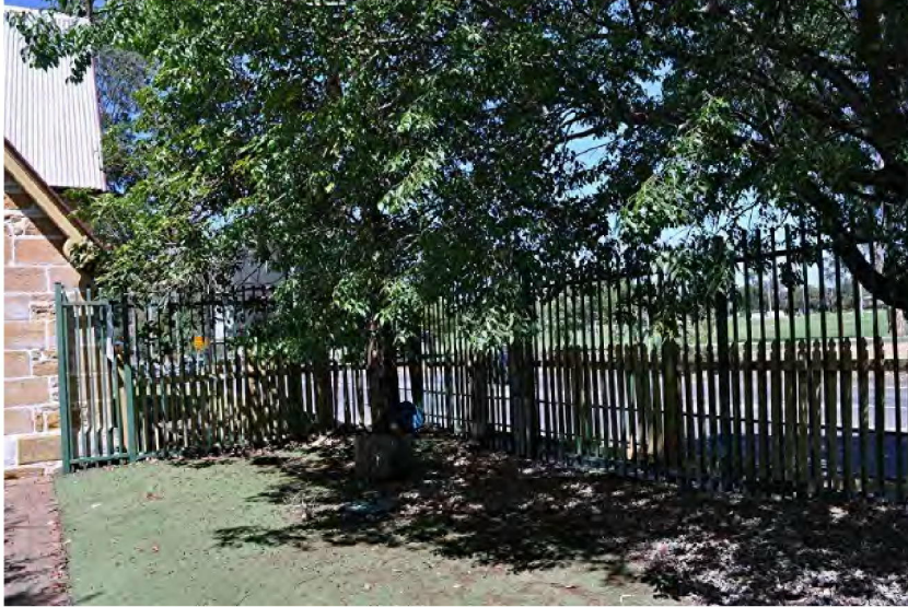
34. Existing fence to the south boundary.
