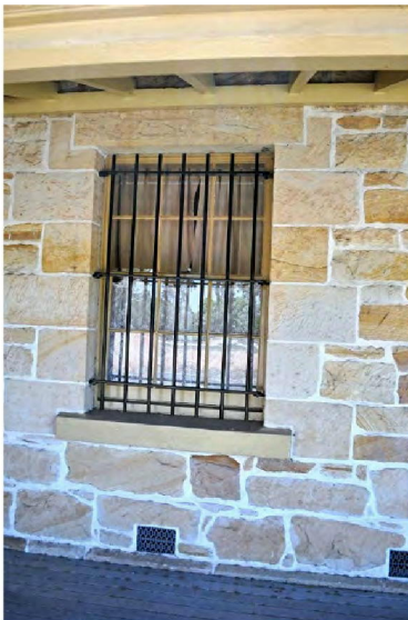
7. West window to south verandah.
