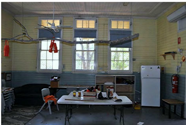
29. Timber schoolroom- west wall.
