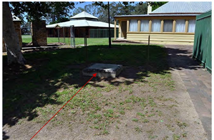
37. Well cap- to the rear of timber classroom.
