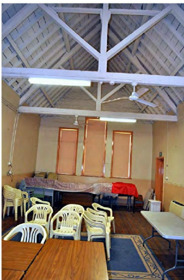
25. Kingpost trusses- schoolroom.
