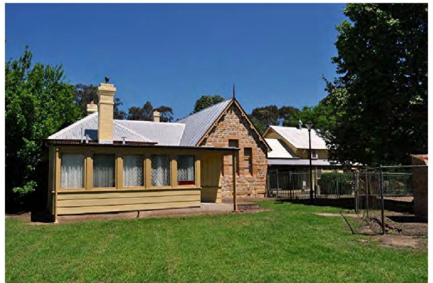
3. Rear of former residence & school (beyond).
