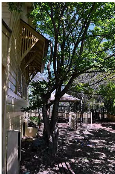
36. Window hood and trough.
