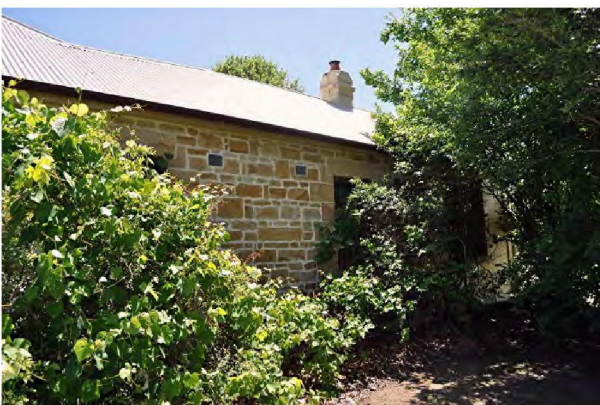
10. East wall of former residence.
