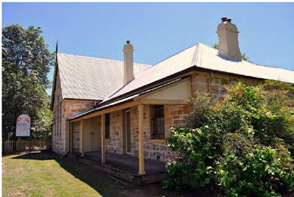
2. Verandah to residence, gable to school room beyond.
