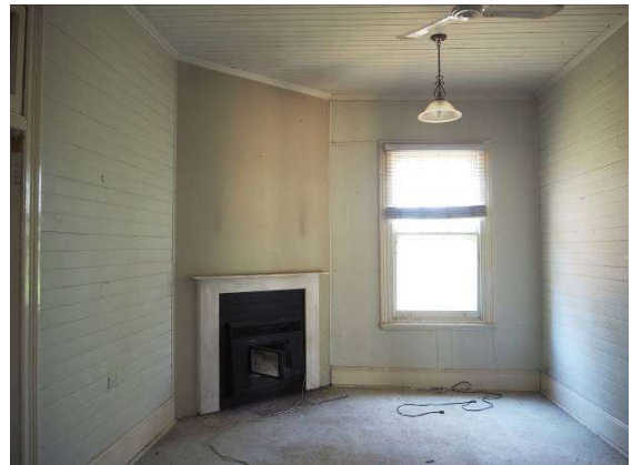
Figure 12: Interior view of existing living room (room 5), looking east.
