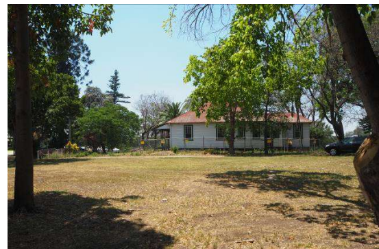
Figure 4: Western elevation of the former Police Station Residence, looking across the adjacent allotments of Nos. 28 and 30 Great Western Highway.
