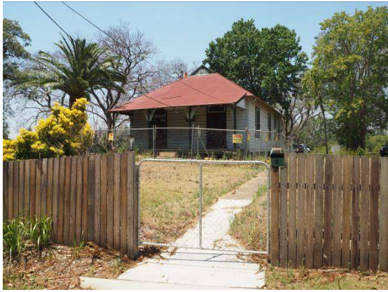
Figure 5: Front (north) elevation of former Police Station Residence.
