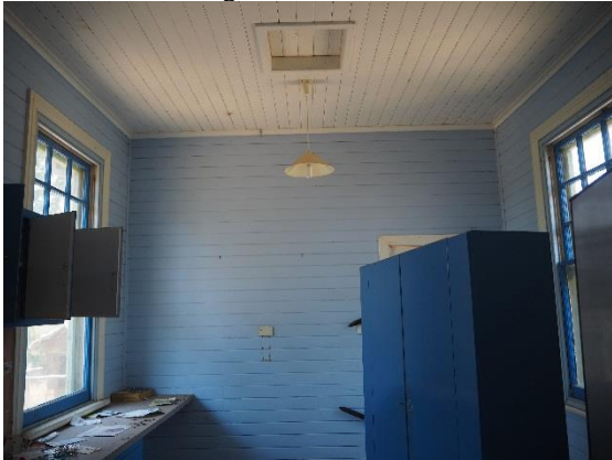
Figure 9: Interior view of existing kitchen looking south (room 8).
