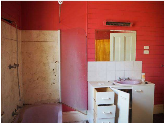
Figure 13: Interior view of existing bathroom (room 4).
