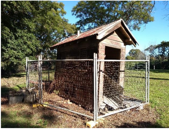
Figure 7: The original weatherboard double privy located in the rear garden of the allotment.
