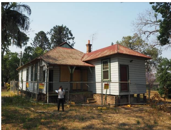
Figure 5: Southern (rear) elevation of the former Police Station and Residence.
