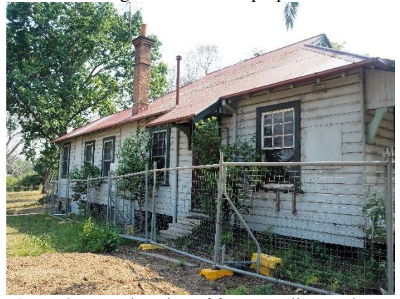
Figure 8: East elevation of former Police Station with original main entry.
