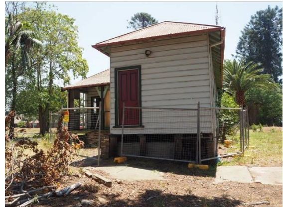
Figure 4: Southern (rear) elevation of the former Police Station and Residence and location of proposed extension.
