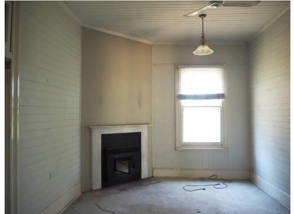
Figure 10: Interior view of existing living room (room 5), looking east.
