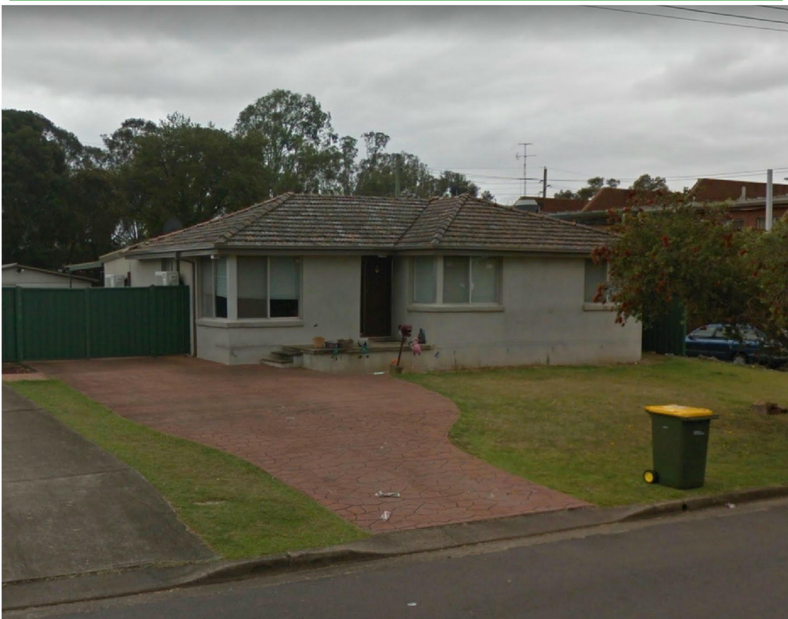
Photograph 1: Shows the subject site – 1 Edna Street
