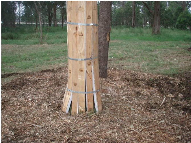
Photo 15: It is flexible for a better fit and is attached using screws to avoid even light impact.
