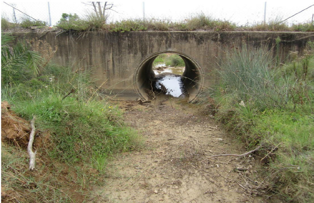
Photograph 1 Drainage construction within east-west channel of the Riparian Corridor
