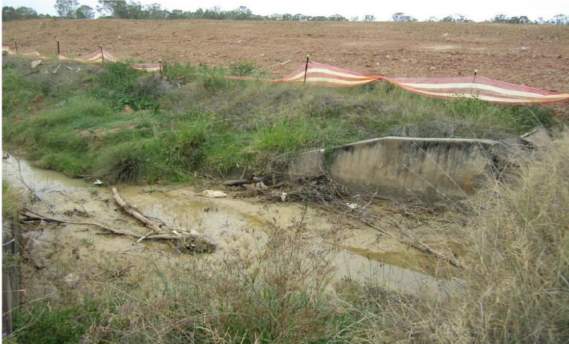
Photograph 2 Cleared drainage pathway within the east-west channel of the Riparian Corridor
