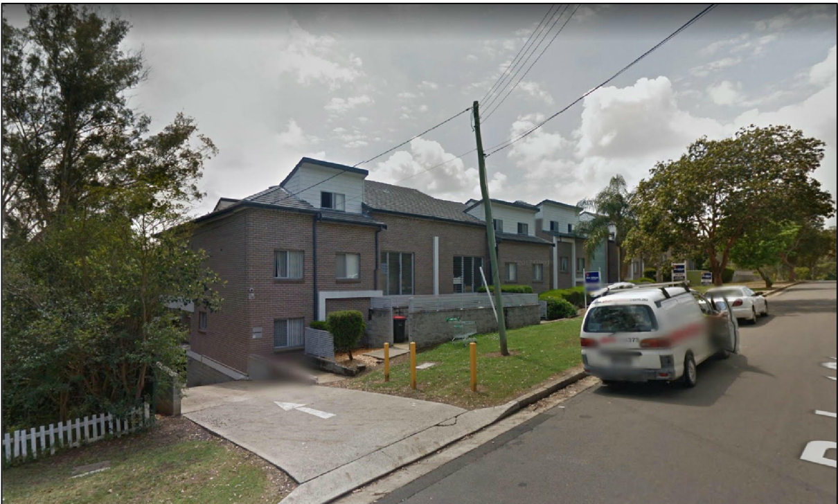
Photograph 2: Shows a recently constructed multi dwelling housing development located opposite the subject site (15-19 Robert Street).
