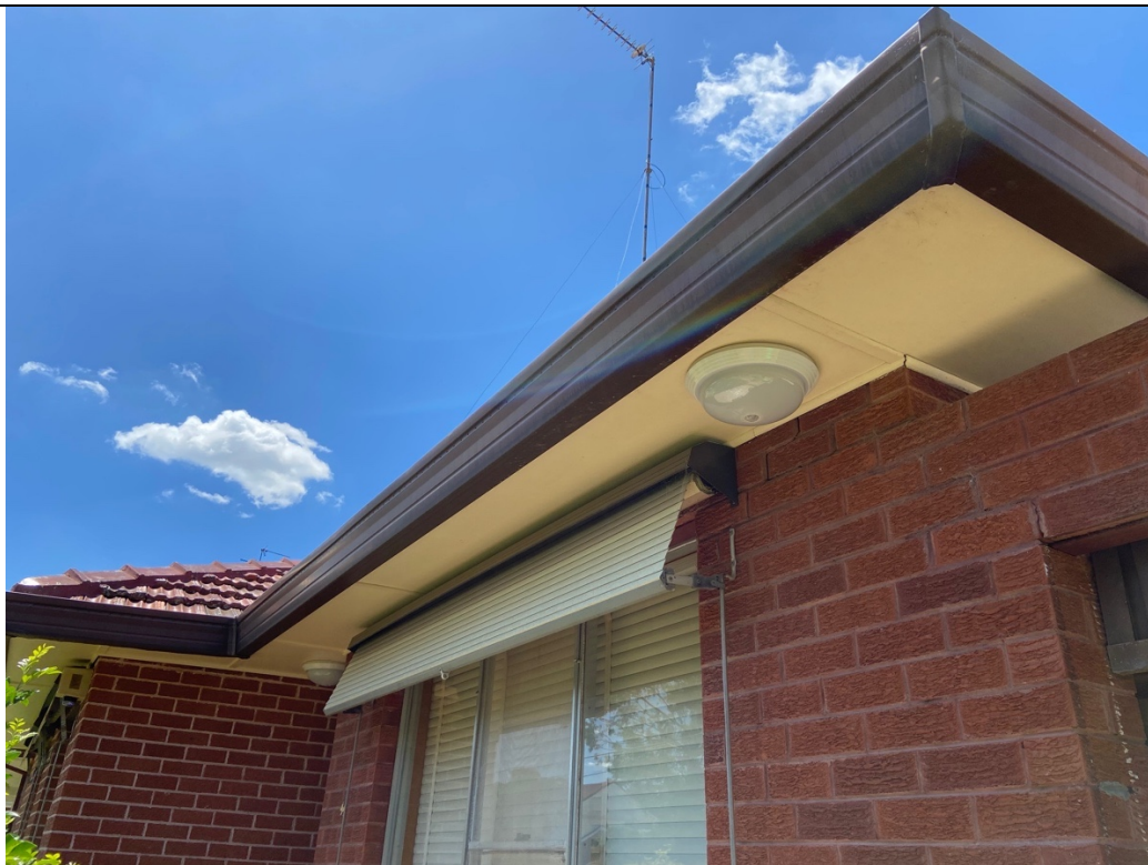
Photo 12 – Suspected Asbestos Containing Building Materials Present to Areas of Built Structures at the Site
