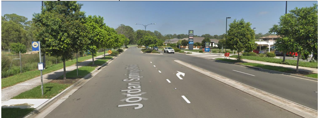
Figure 8 – Jordan Springs Boulevard, westbound (Source: Google maps)
