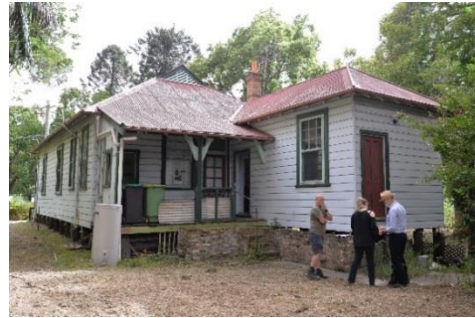
Figure 4: Southern (rear) elevation of the former Police Station and Residence.
