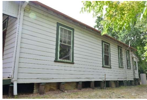
Figure 8: West elevation of former Police Station with original main entry.
