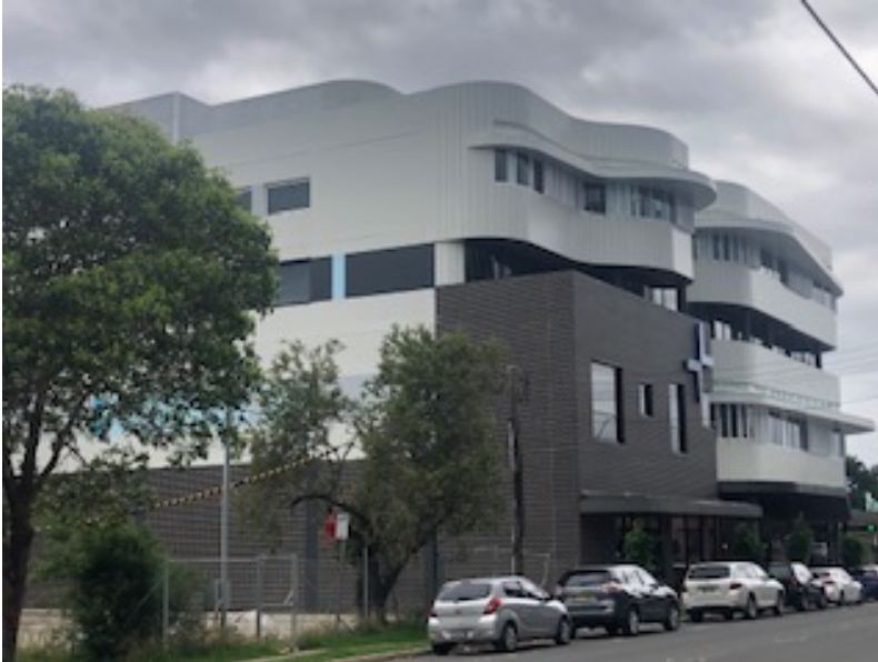
Figure 7. Somerset Specialist Centre at 28-32 Somerset Street, Kingswood
