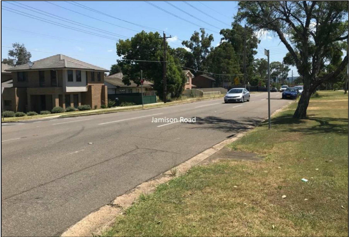
Figure 2-6: View looking west along Jamison Road
