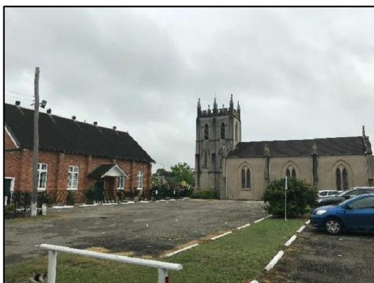
Figure 22. Heritage item in the vicinity of the subject site (St. Stephens Church and hall from rear)
