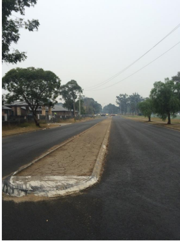
Photo 5. Looking west along Boronia Road. The subject site is to the right of picture.
