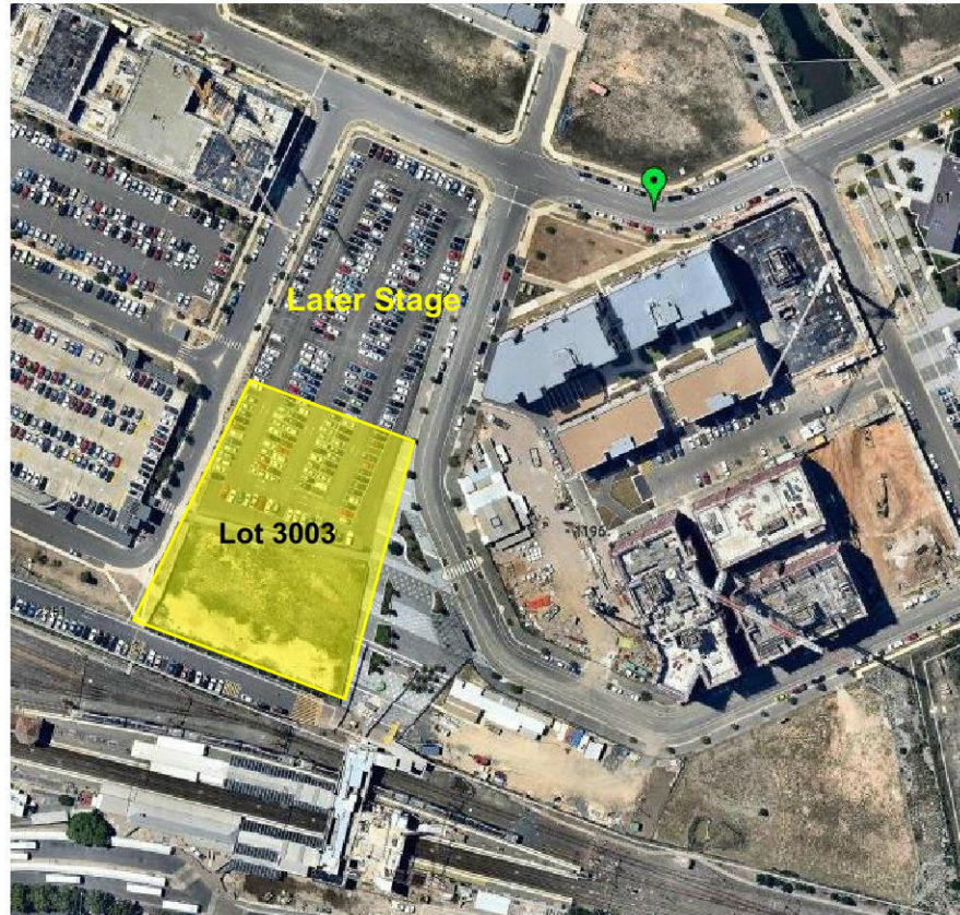
Photograph courtesy of NearMap
