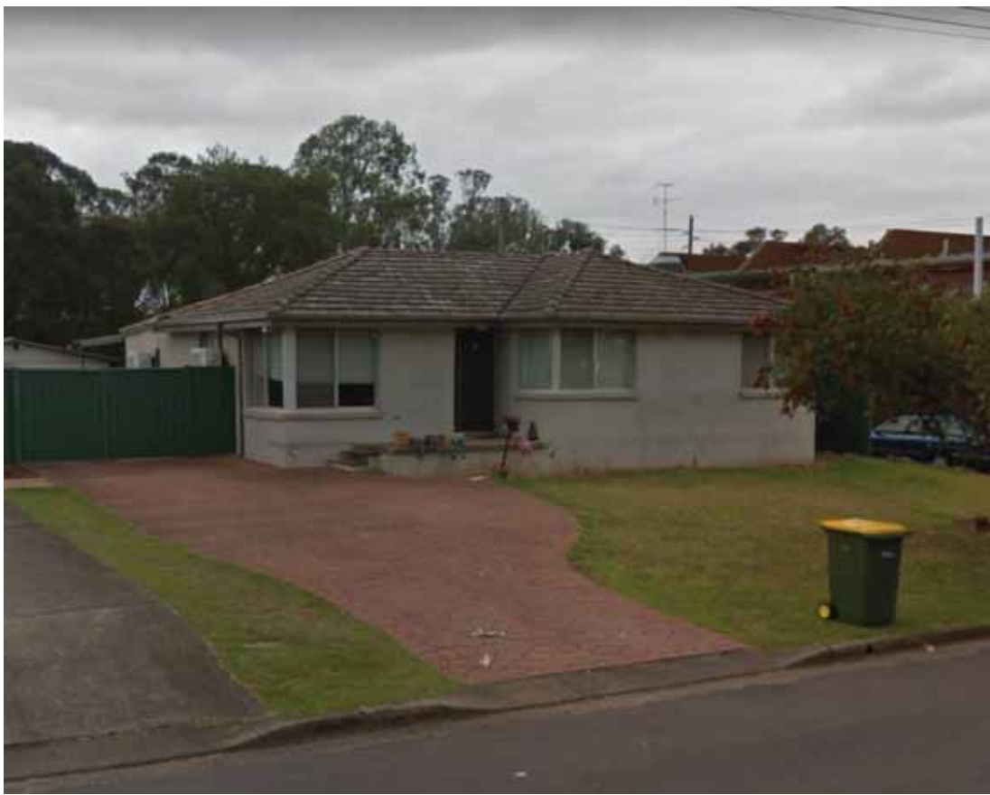
Photograph 1: Shows the subject site – 1 Edna Street
