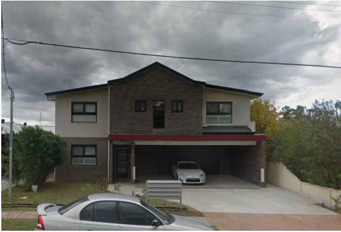
Photograph 2: Shows a recently constructed comparable boarding house No. 55 Second Ave, Kingswood
