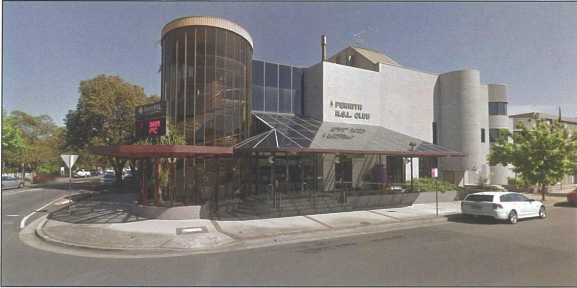
Existing Castlereagh Street entrance to the RSL Club to be retained
