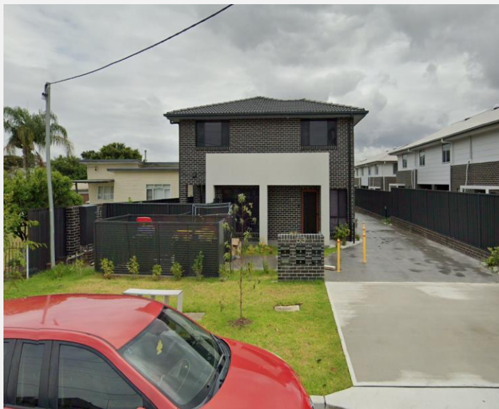
Nearby multi dwelling housing development
