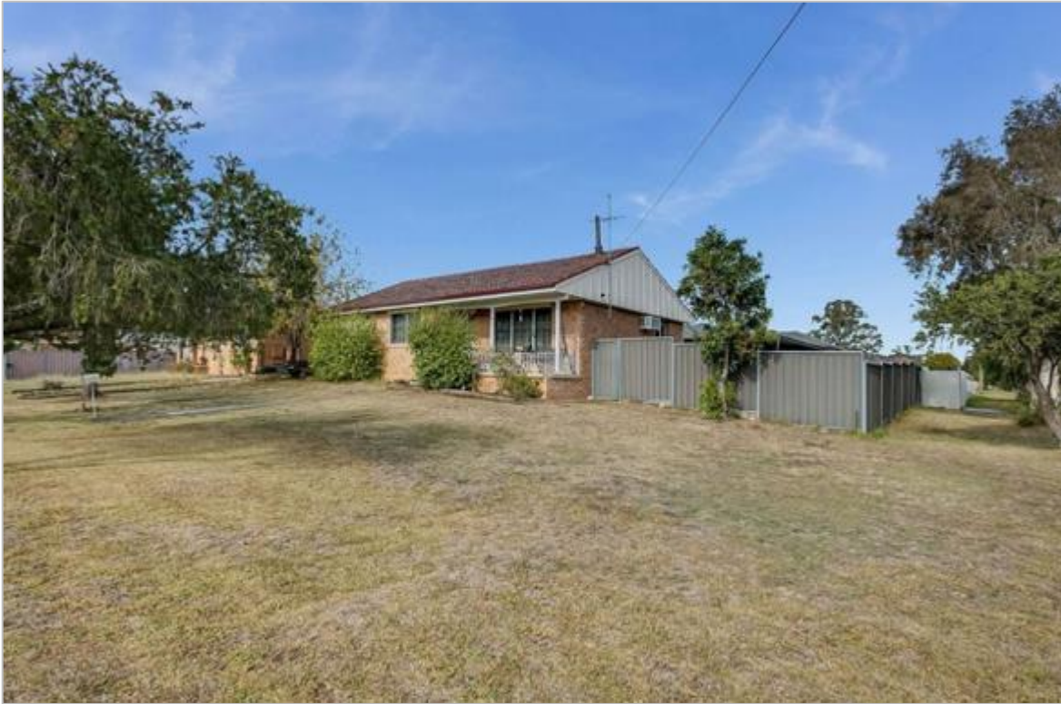
Figure 3: Existing built form
