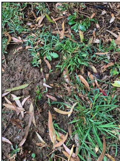
Figure 7: Showing heaving soil around the base of Tree 8.
