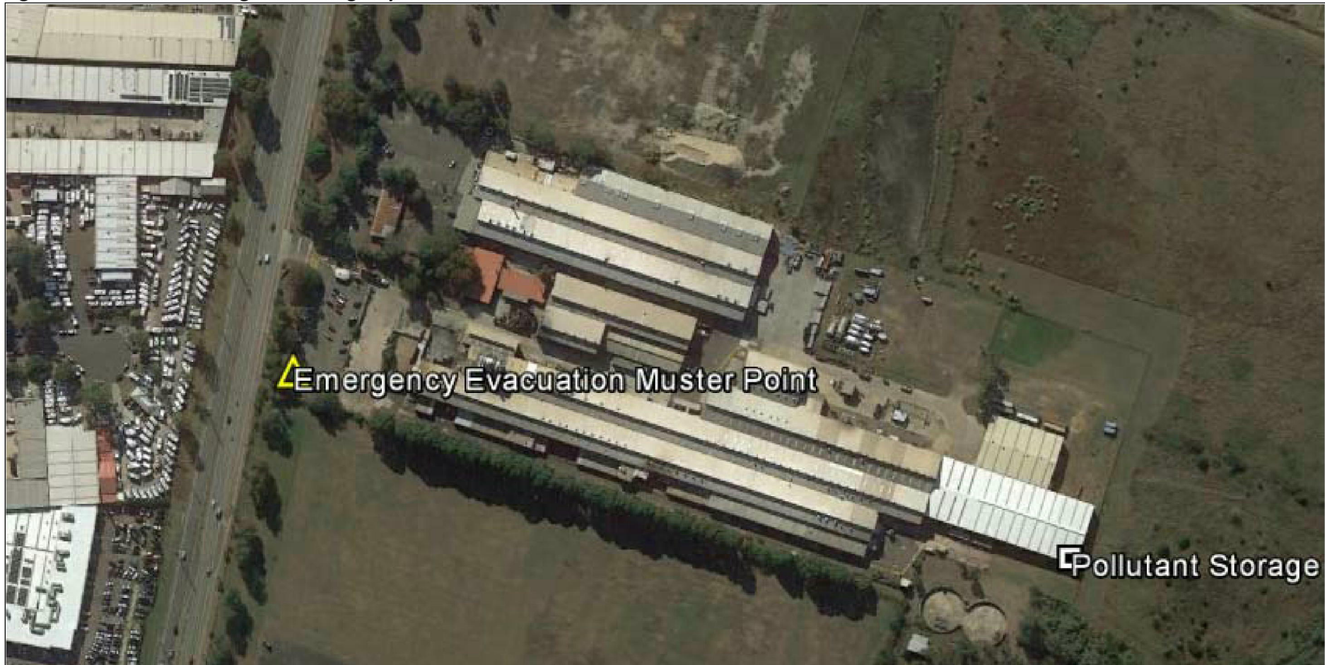
Figure 10.2. Pollutant Storage and Emergency Evacuation Muster Point.
