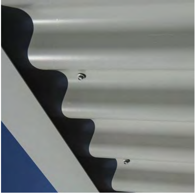
CLD-3 SOFFIT LINING Lysaght Custom Orb Profile - Shale Grey
