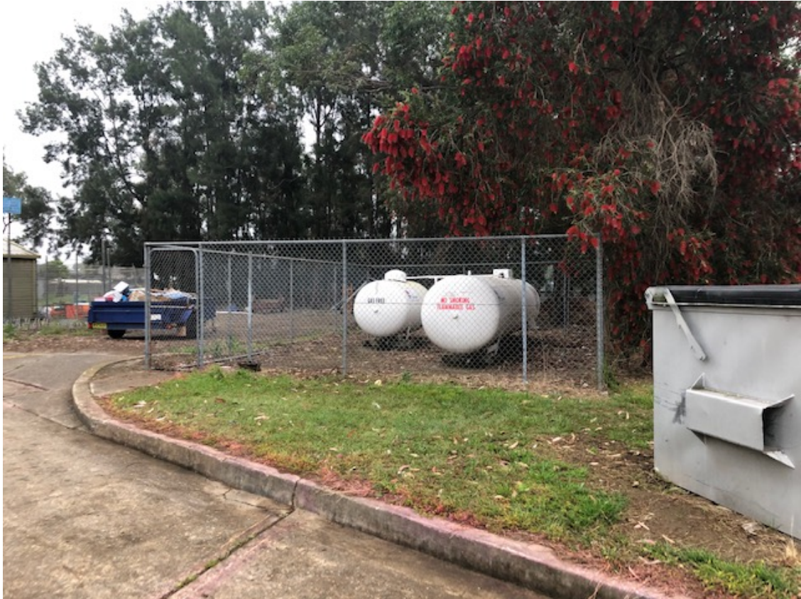
Plate 3 View looking north-west – gas tanks to be removed
