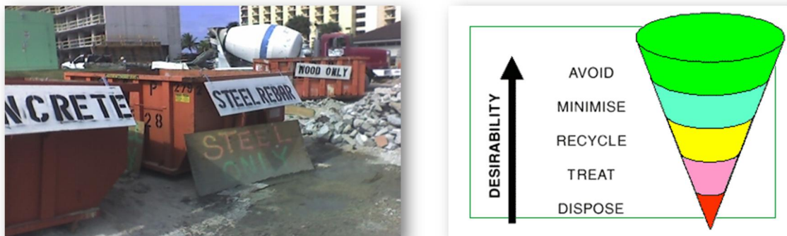
Figure 10 Implement construction waste management practices on-site
