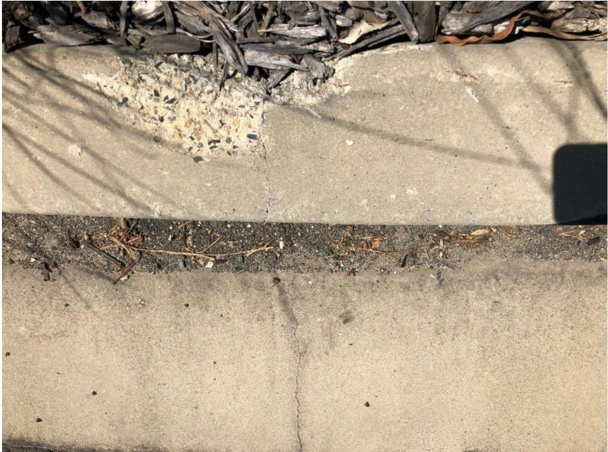
*Figure 79: chip to top of kerb.*
