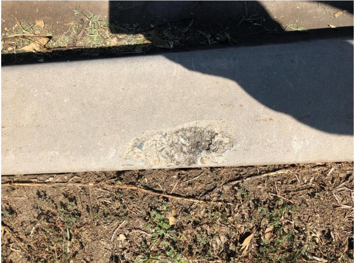
*Figure 75: chip to top of gutter.*
