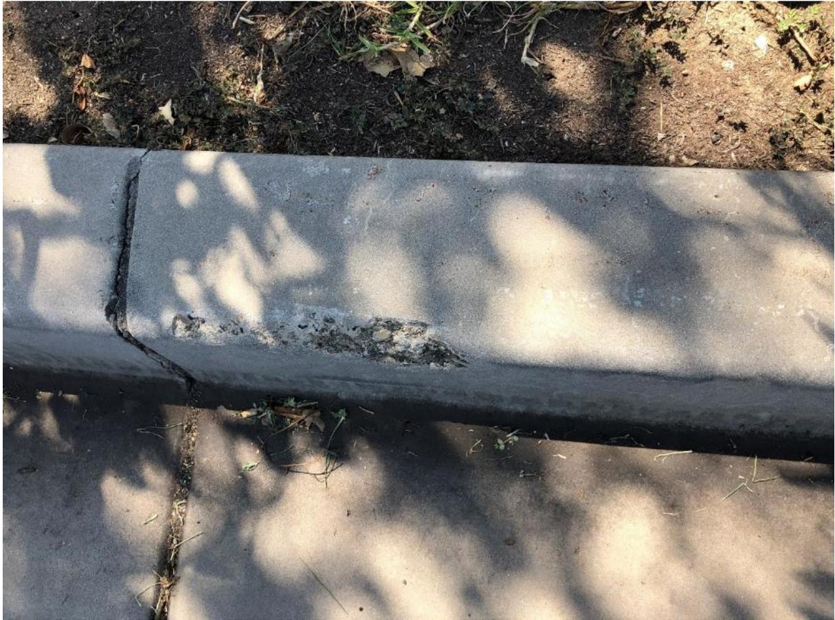
*Figure 74: chip to top of gutter.*
