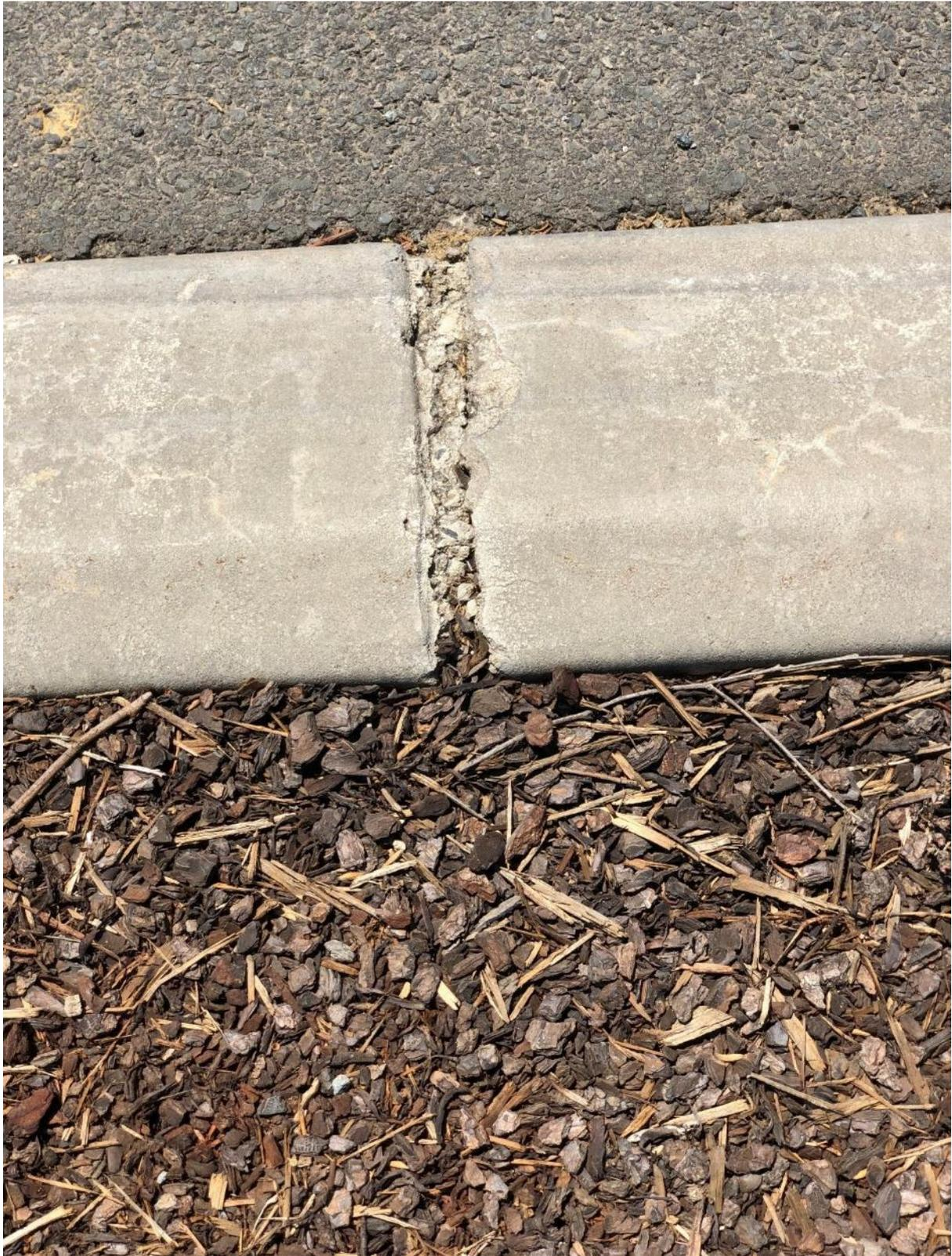
*Figure 18: separation of median strip kerb.*
