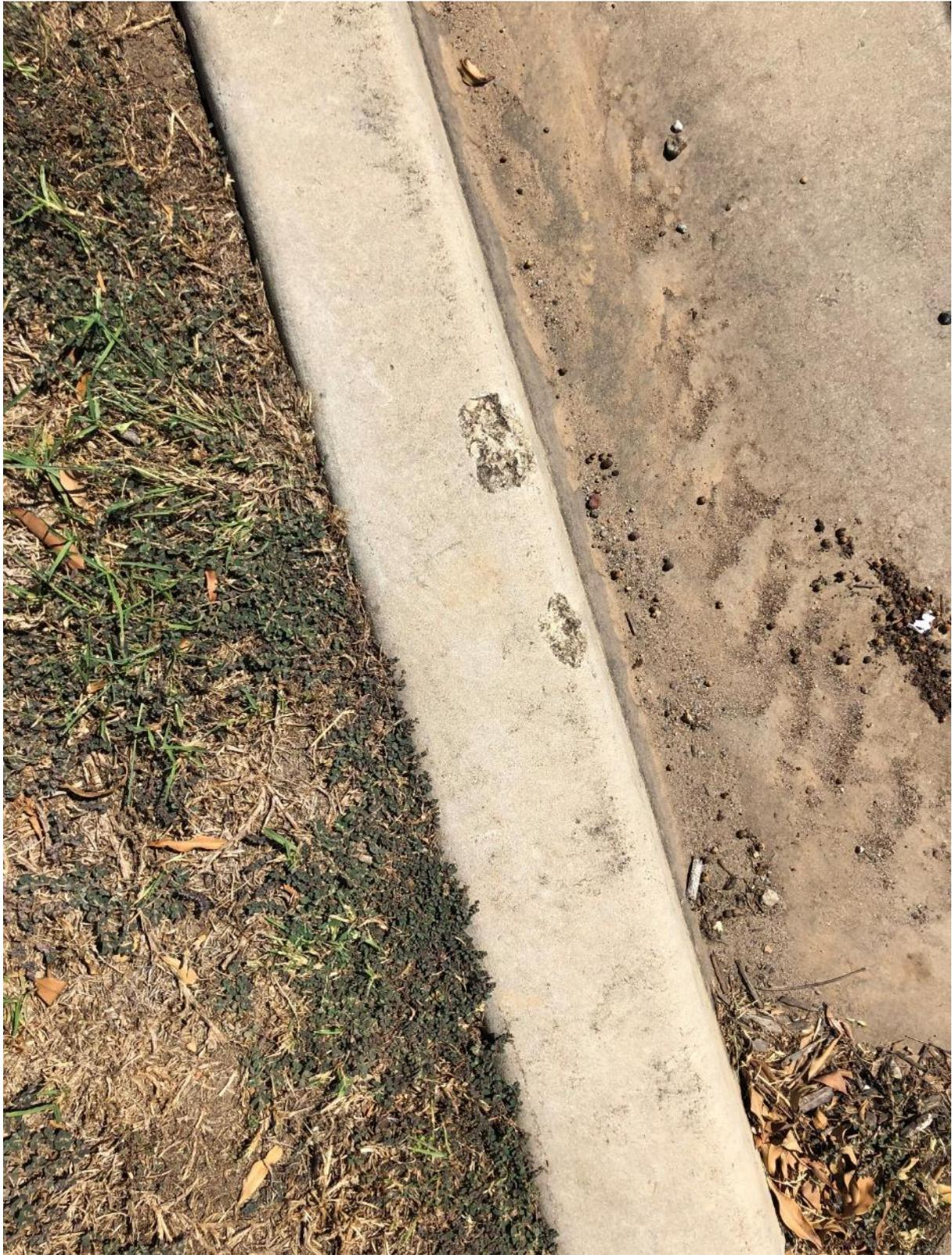
*Figure 41: chips on top of kerb.*
