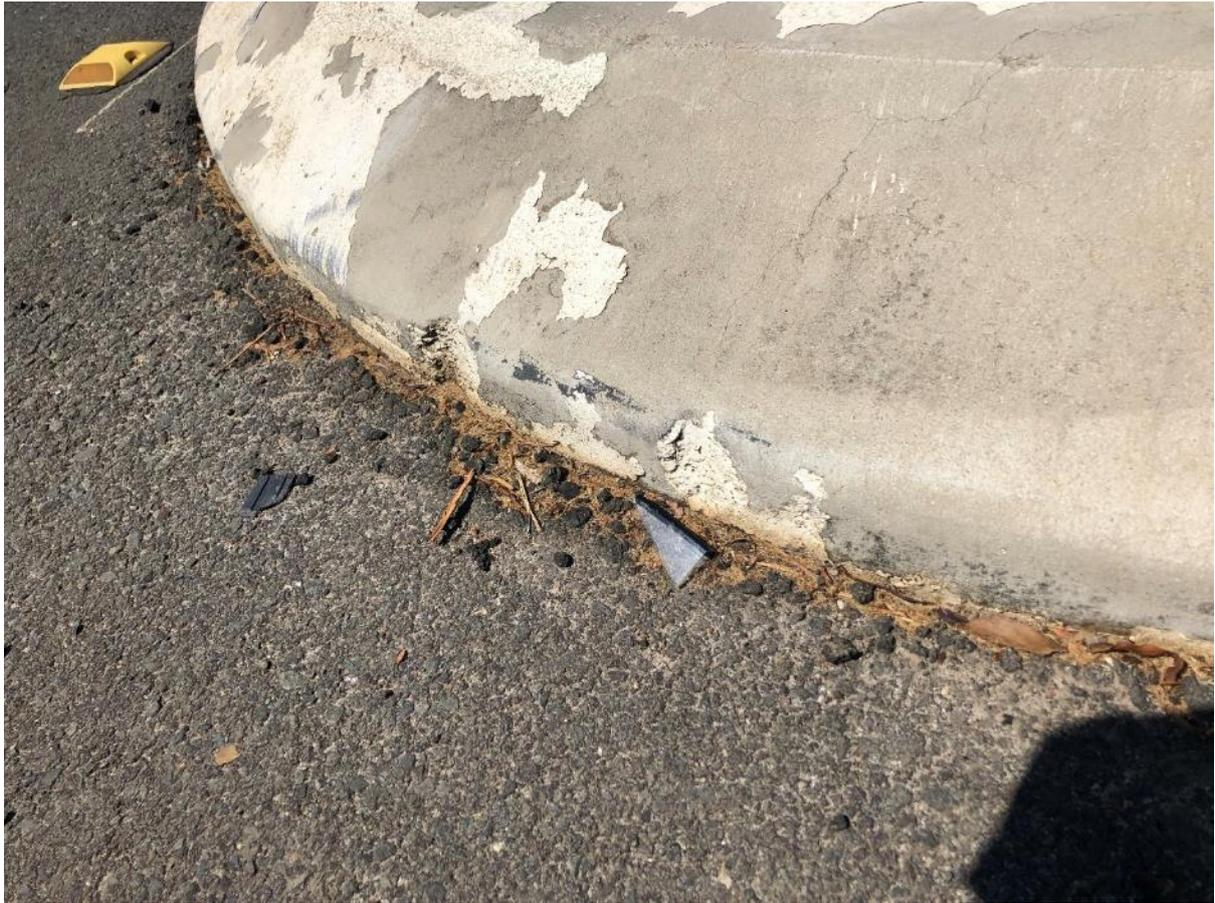
*Figure 1: chips in median strip kerb (facing The Northern Road)*
