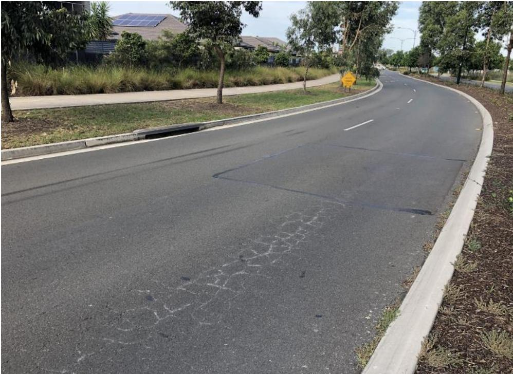
Figure 89: Approx CH255 EB Pavement failure
