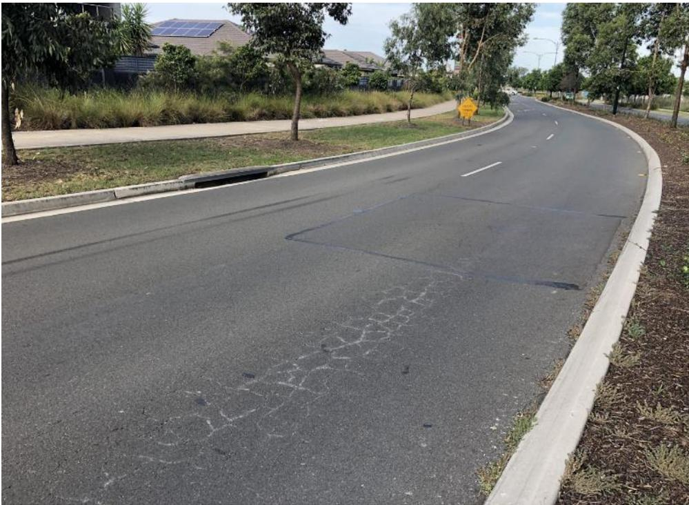
Figure 89: Approx CH255 EB Pavement failure
