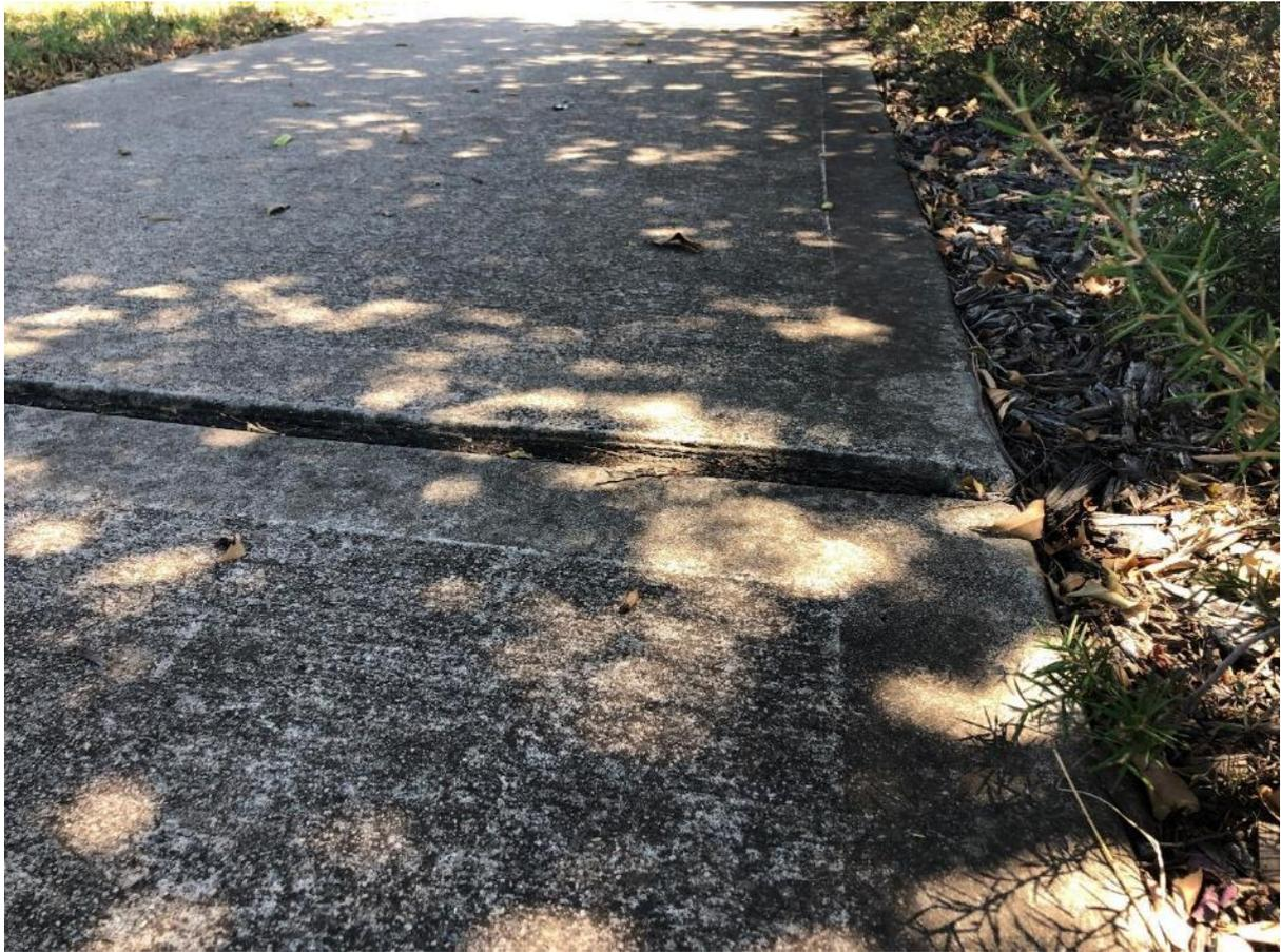
*Figure 84: footpath bay lifted at expansion joint interface.*
