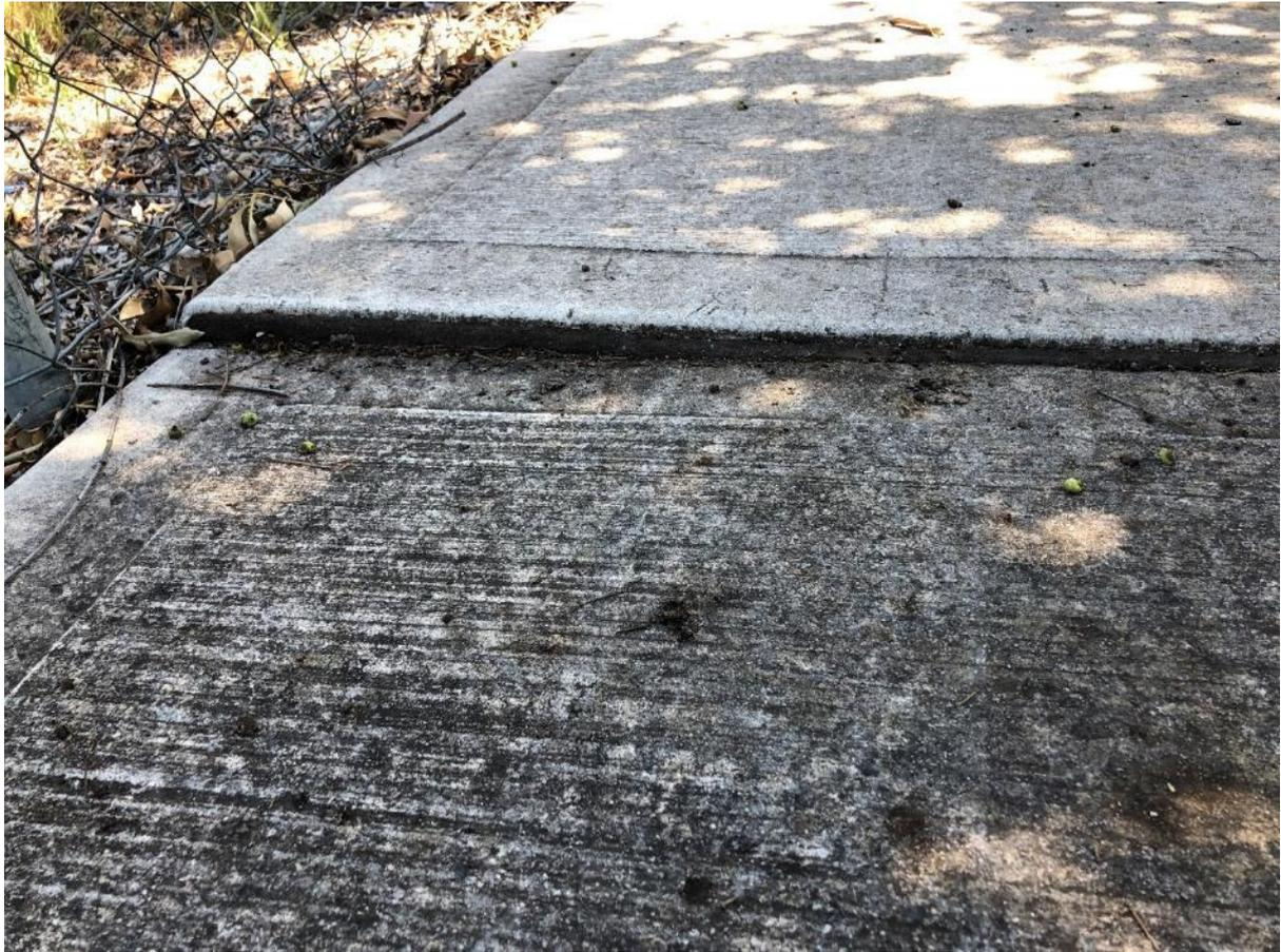
*Figure 87: footpath bay lifted at expansion joint interface.*
