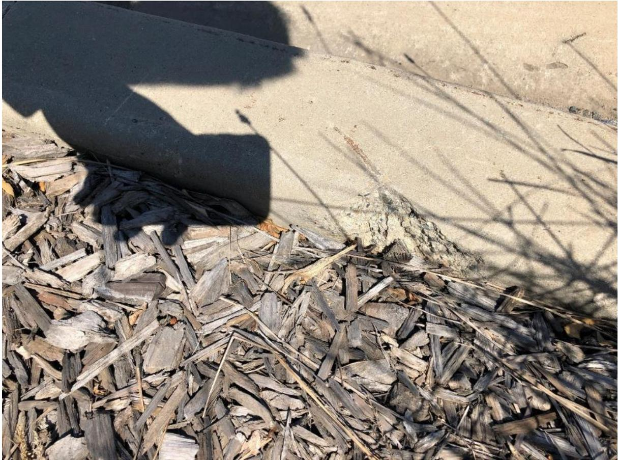
*Figure 80: chip to top of kerb.*
