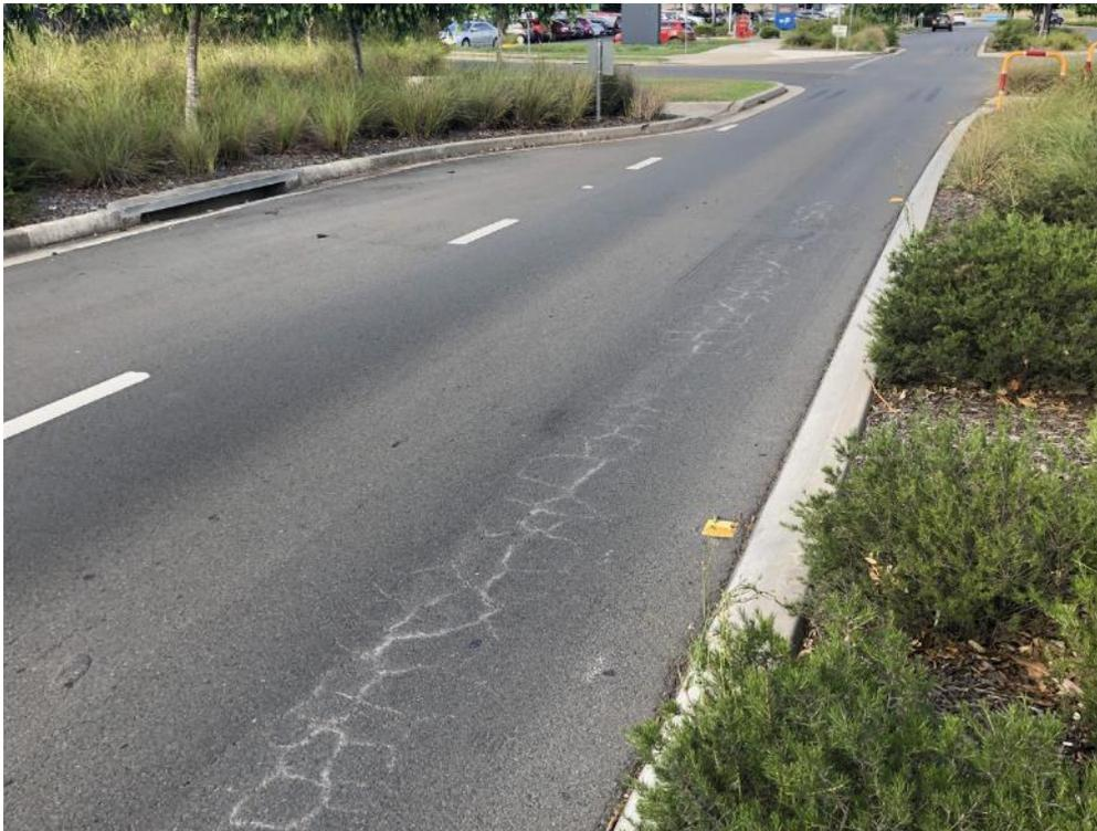
Figure 91: CH330 EB pavement failure at wheel track (P72)
