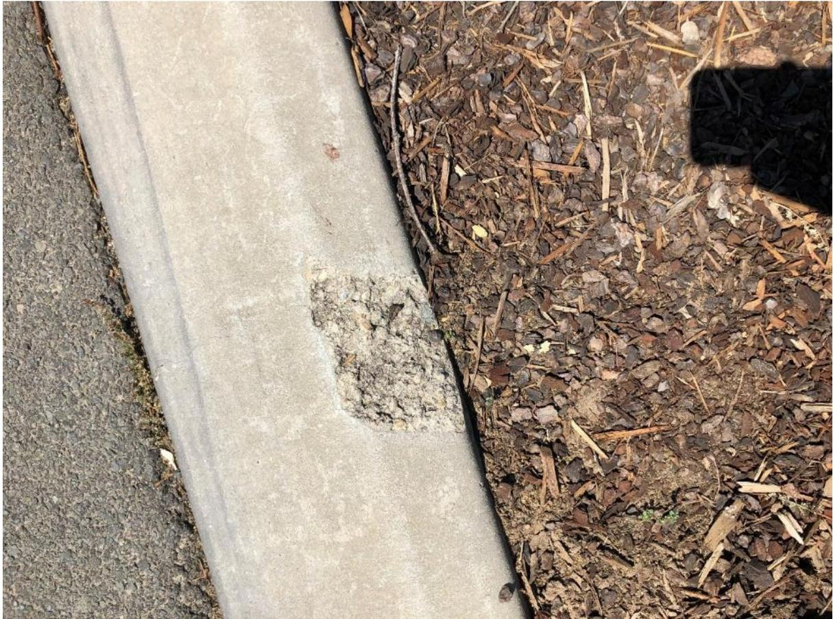
*Figure 19: chip on top of median strip kerb.*
