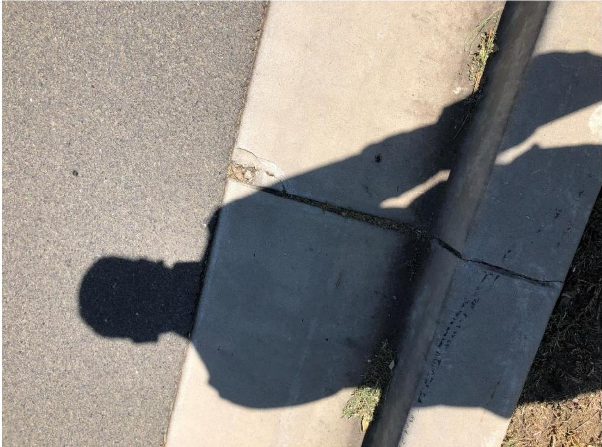
*Figure 72: chip to gutter at construction joint interface.*
