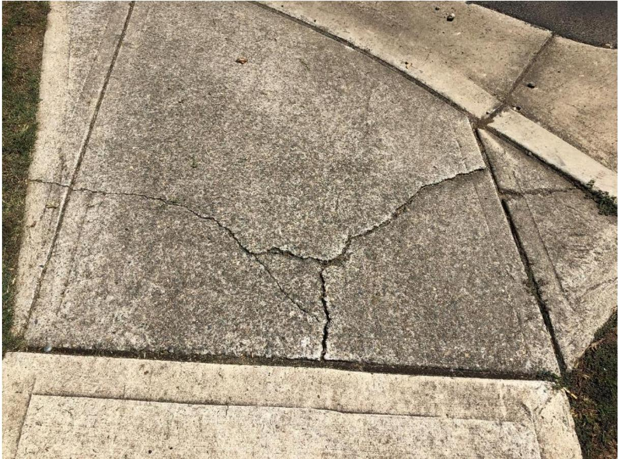
*Figure 85: cracking to pram ramp located left of proposed site entry.*
