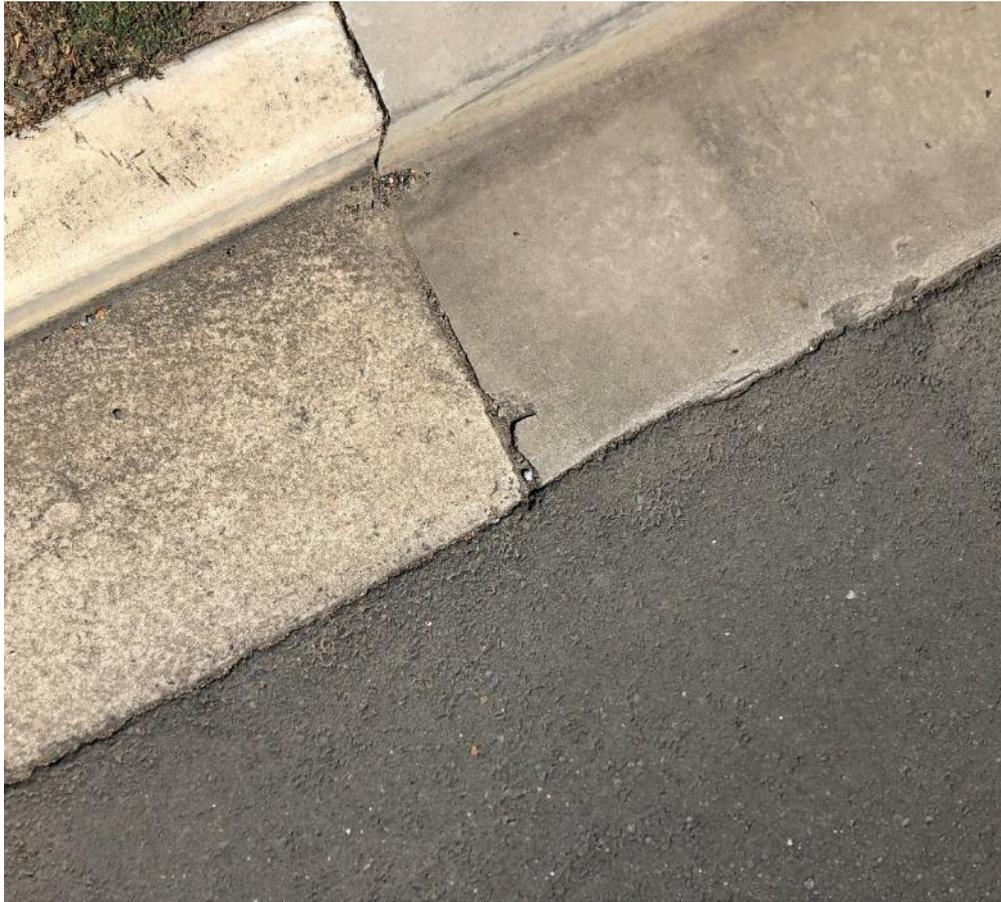
*Figure 42: spalling on edge of construction joint interface on gutter.*
