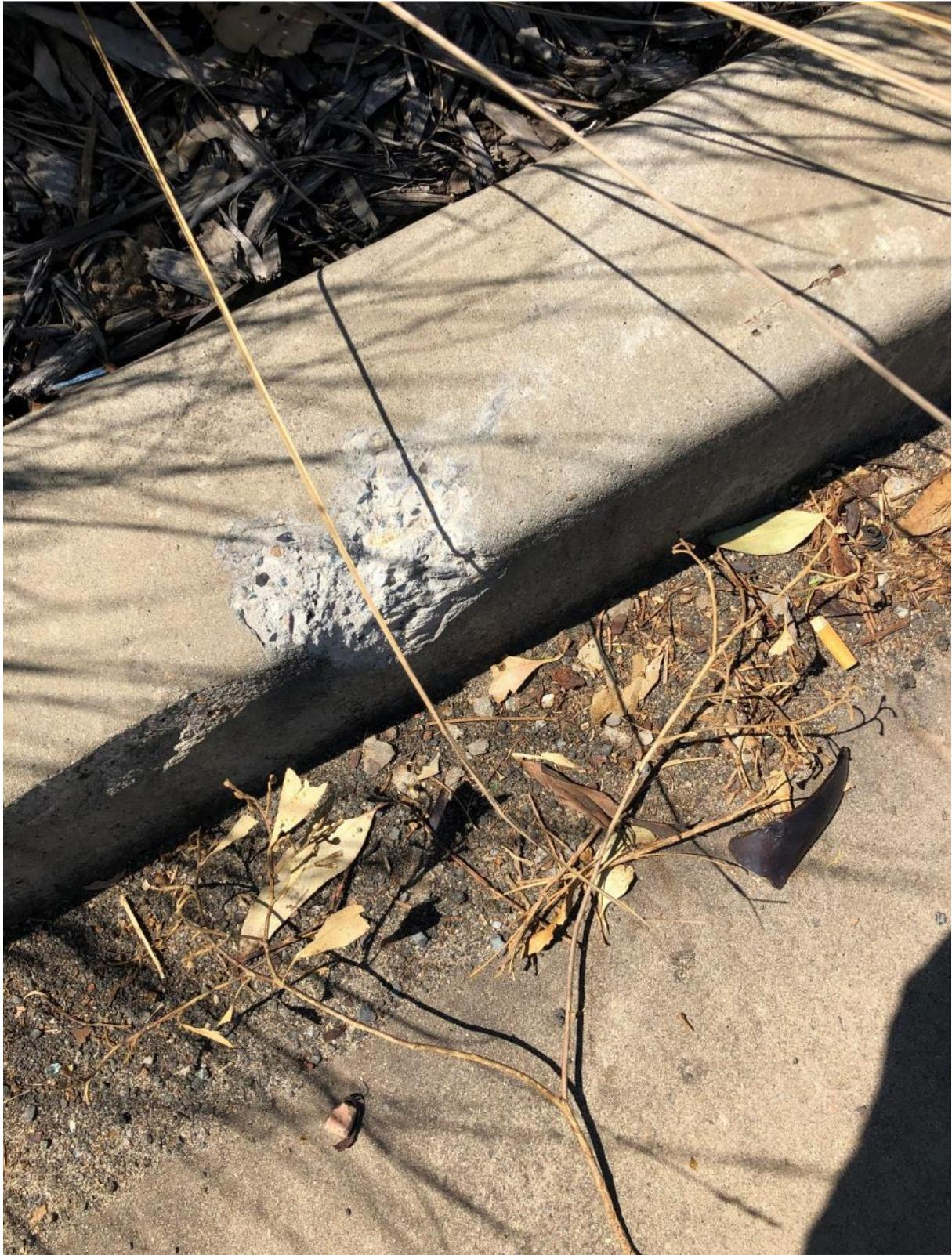
*Figure 78: chip to top of kerb.*
