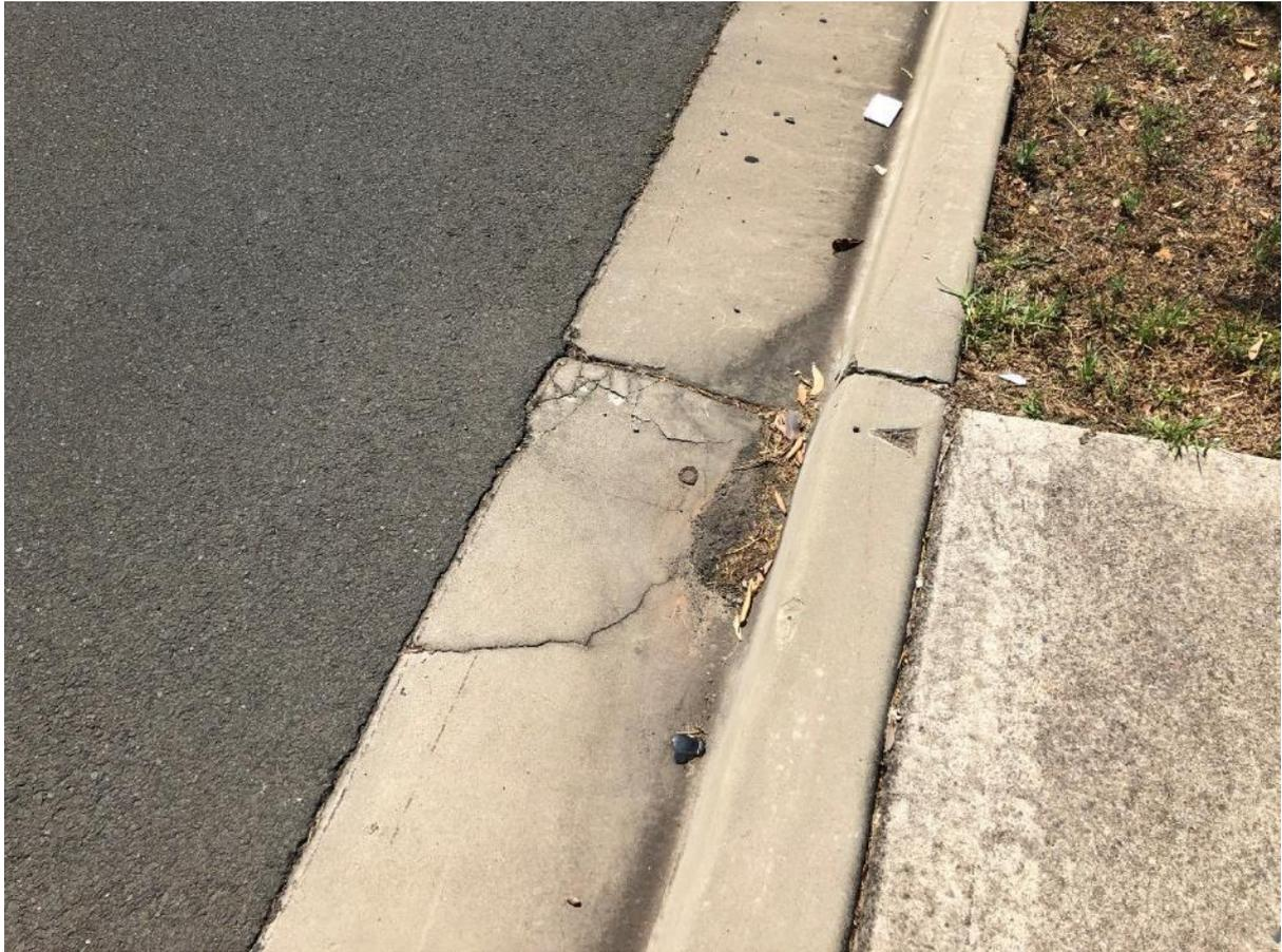
*Figure 83: cracking to gutter, adjacent to top of left wing.*
