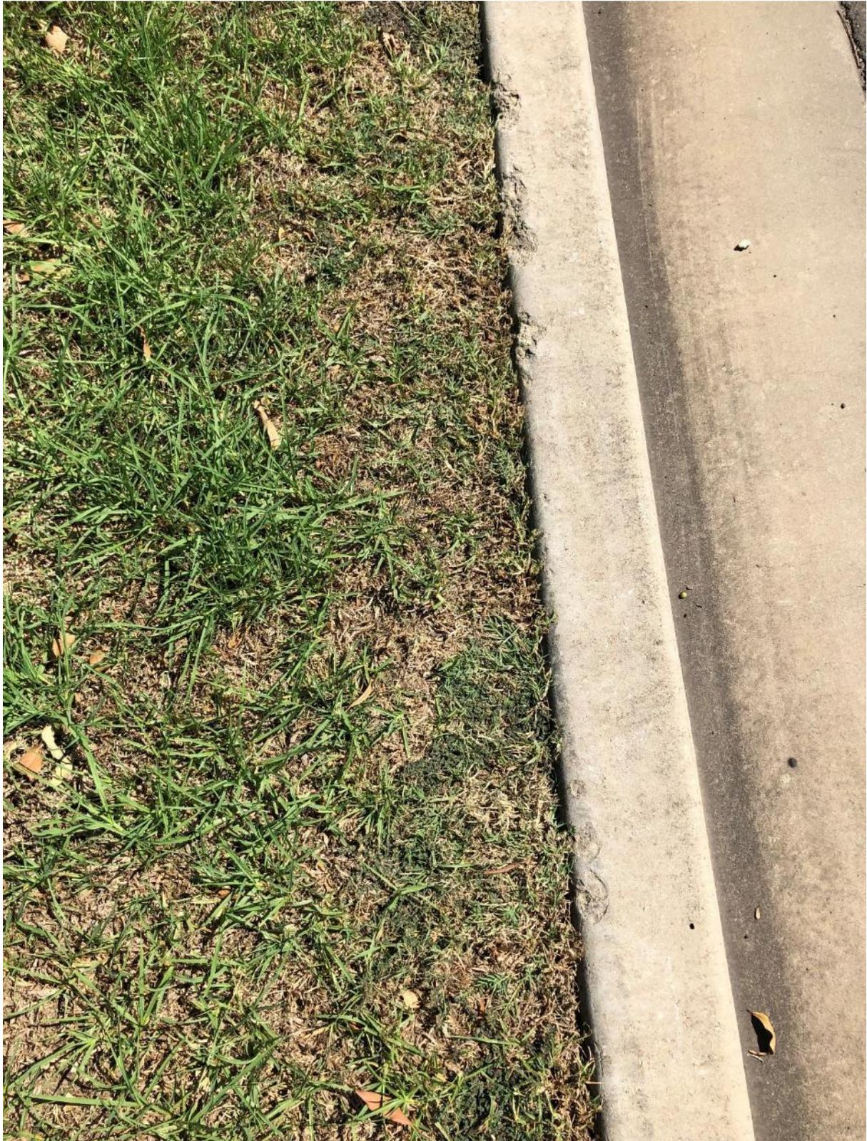
*Figure 40: chips to top of kerb and gutter.*
