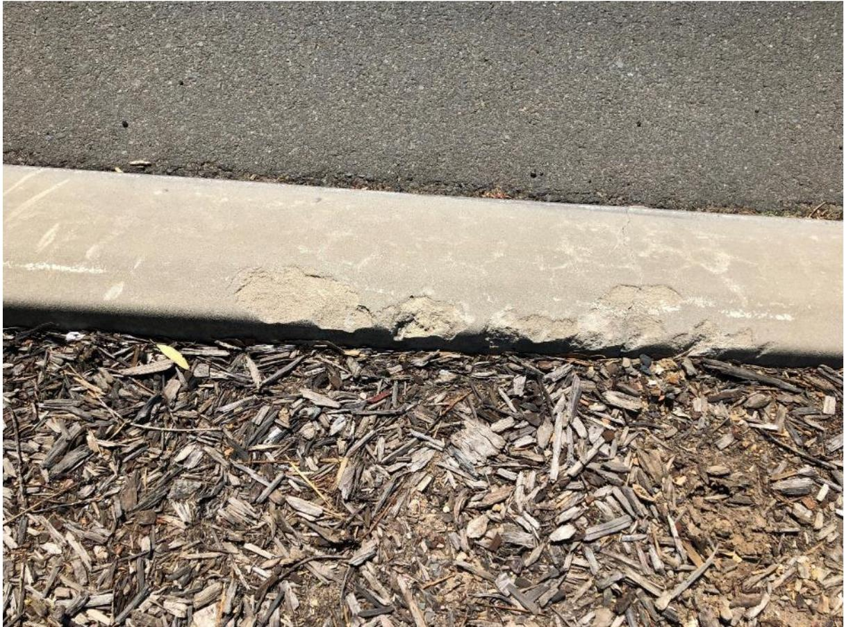
*Figure 20: chips on top of median strip kerb.*
