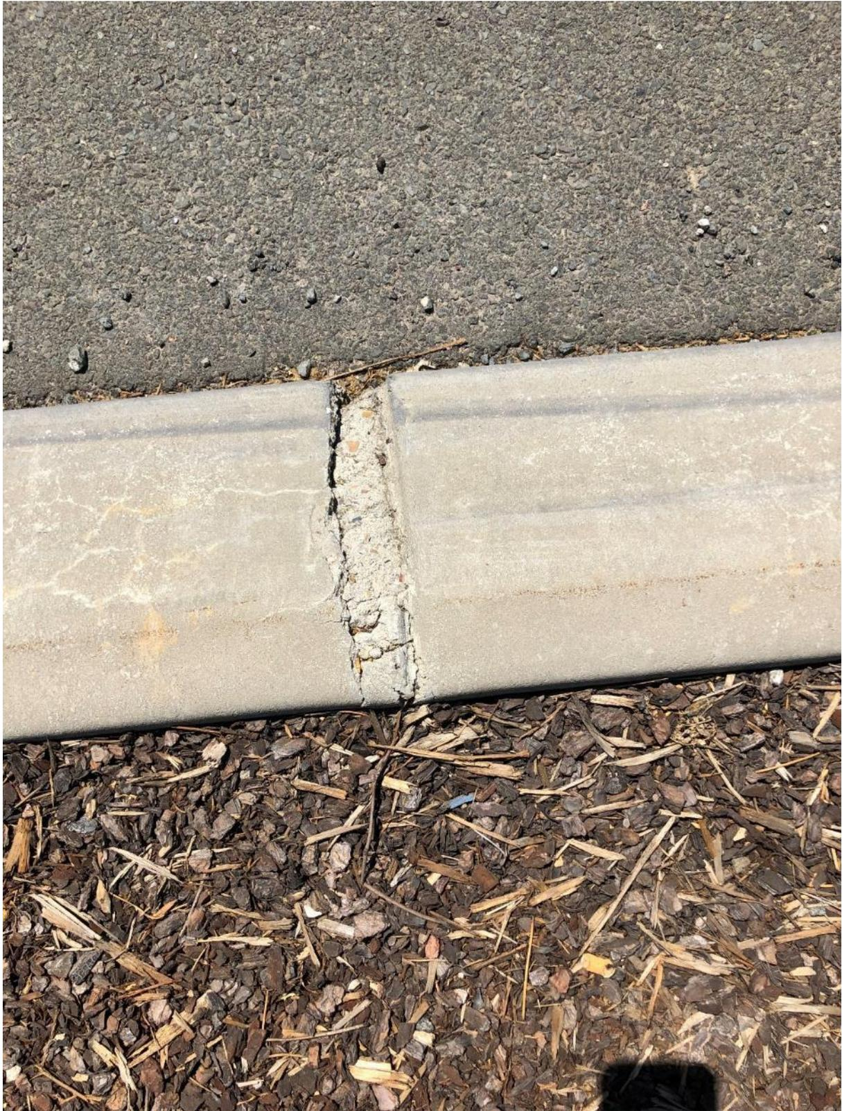
*Figure 17: separation of kerb at construction joint interface.*
